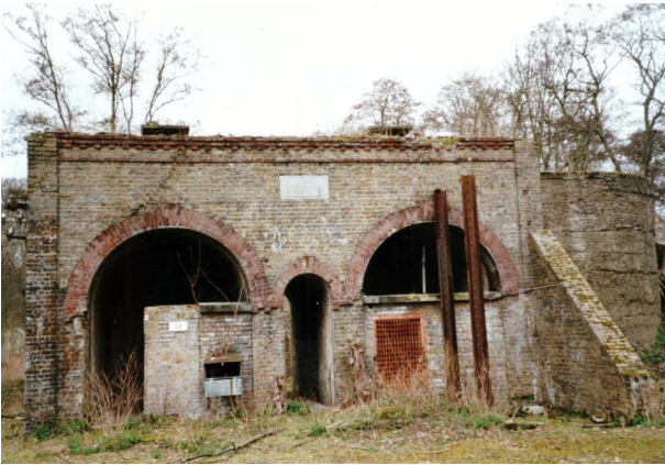
S31 Entrance tunnel and two Bays 1994
