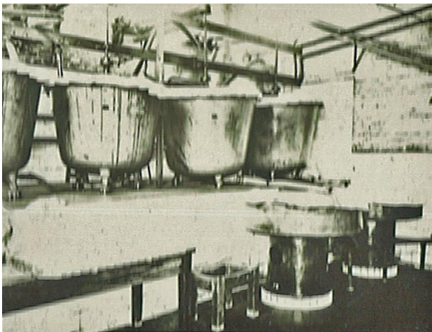
CE Purification Plant Acetone Stills
