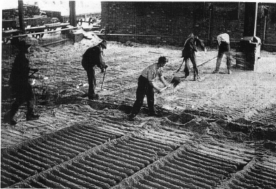
This picture shows the casting of pig iron in a traditional pig bed at Lifford Hill Furnace in Shropshire. I have included it simply because such a sight (it was most impressive) will never be seen again. Pig iron is still made, but it is all machine cast now.
