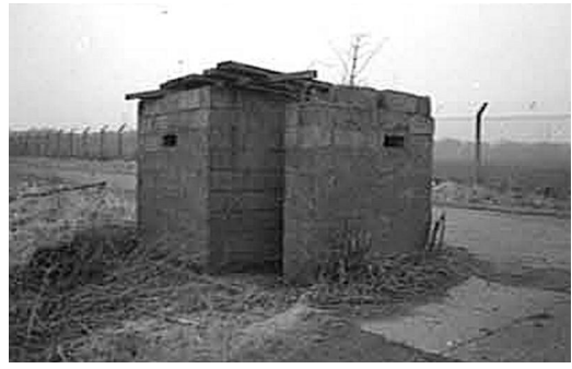
S43 Police Gate House
