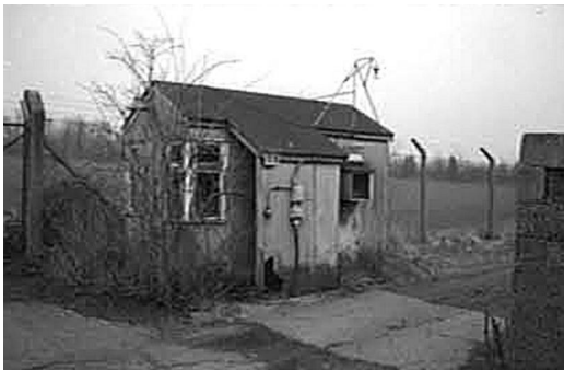
S9 Police Gate House
