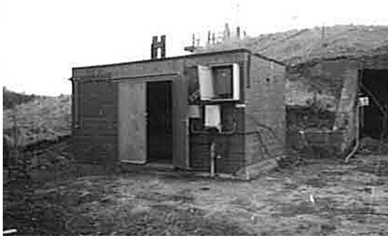
S15 1941 Plenum Heater House 195? FP 1 Control Room
