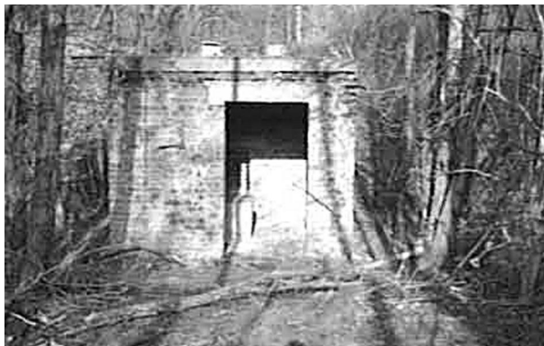
S22 1941 Plenum Heater House 195? FP2 Control room
