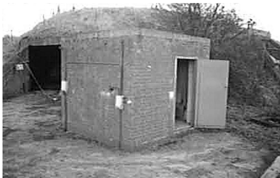
S17 1941 Expense Magazine 195? FP 1 Control Room
