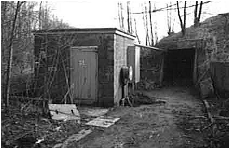
S20 1941 Plenum Heater House 195? FP2 Control Room
