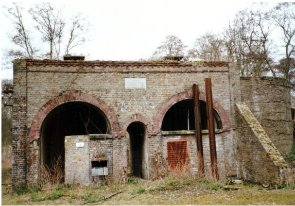
S31 Entrance tunnel and two Bays 1994
