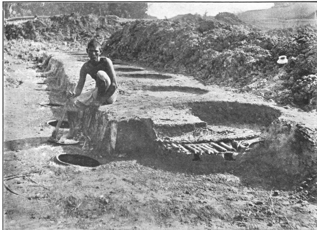
FIG. 3. Percolators for Extracting Indian Crude Saltpetre.
