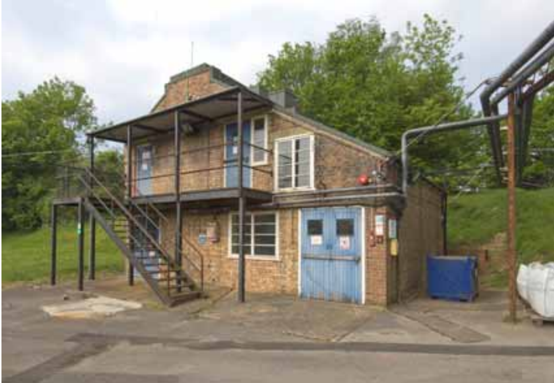
Figure 4: Experimental filling shed F11 erected in 1938 for filling cordite rocket motors. © English Heritage DP060536
