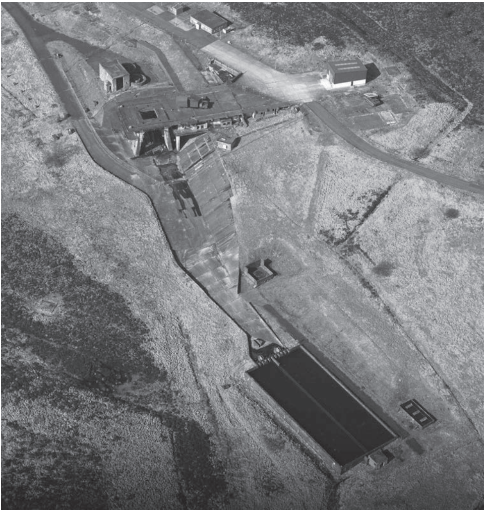
Fig. 15 Spadeadam, Cumbria, Greymare Hill, C3 test stand, flume and effluent settling pool, scheduled. (© Historic England 17819/16)
