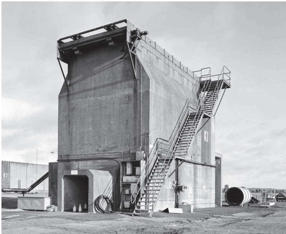
Fig. 9 Westcott, Buckinghamshire, stand K1 for firing inverted motors, Listed Grade II. (© Historic England BB94/04860)
