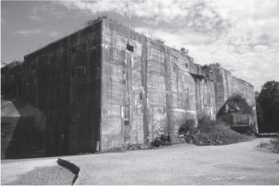
Fig. 31 Eperlecques, Northern France, the massive bunker built for the assembly and launch of V2 rockets. Construction began in 1943, but was halted by allied bombing. (© Wayne D Cocroft)
