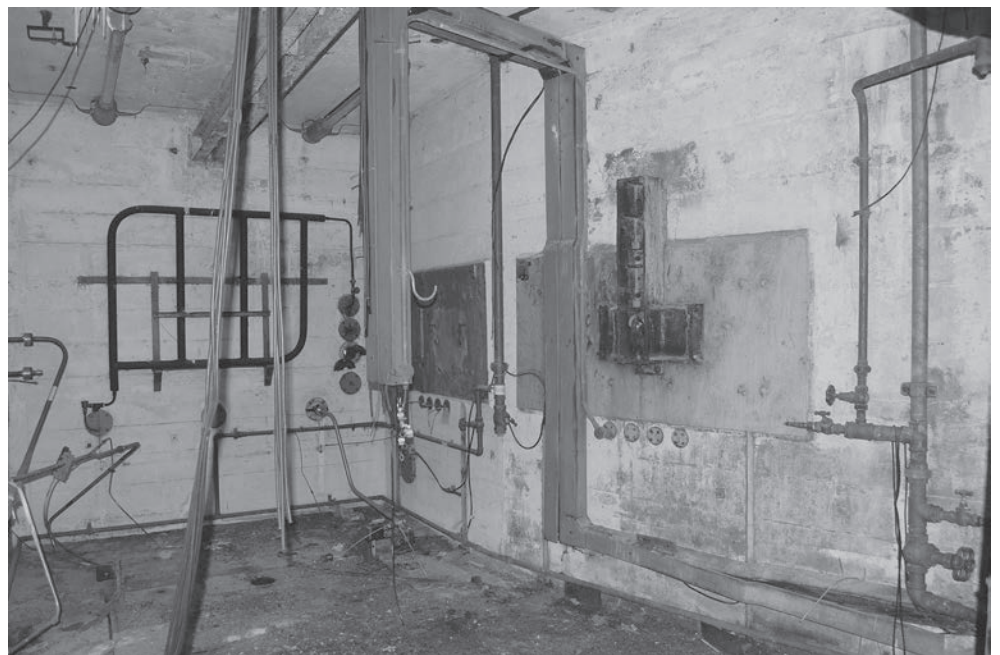
Fig. 8 Westcott, Buckinghamshire, Stand C, showing the observation window openings blocked after the 1947 explosion. (© Wayne D Cocroft)
