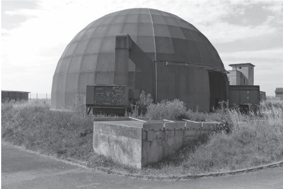
Fig. 25 RAF Kirton in Lindsey, Lincolnshire, Rapier training dome used to practice tracking targets. (© Wayne D Cocroft)
