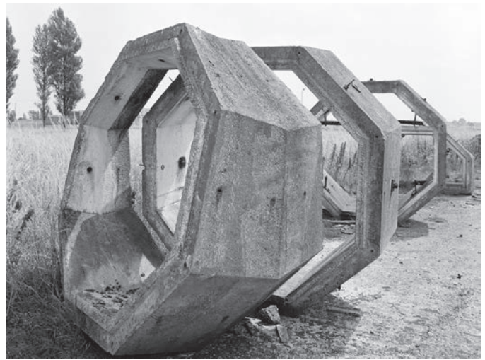
Fig. 17 Westcott, Buckinghamshire, sections of the one sixth scale underground launcher model. (© Historic England BB99/04750)
