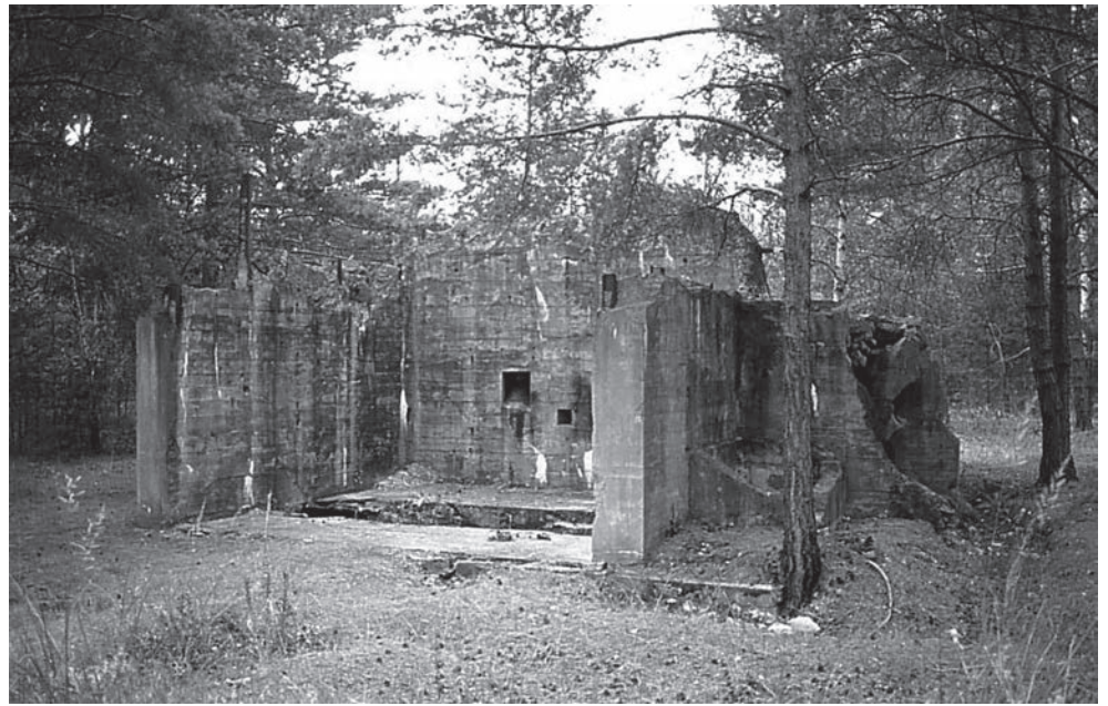
Fig. 6 Kummersdorf, Brandenburg, it was in this test stand that Werner von Braun undertook his phd research. The design of the with separate fuel and oxidant bays, water-cooled efflux ducts, and an adjacent control and direct observation room set the basic design for many subsequent test stands. (© Wayne D Cocroft)
