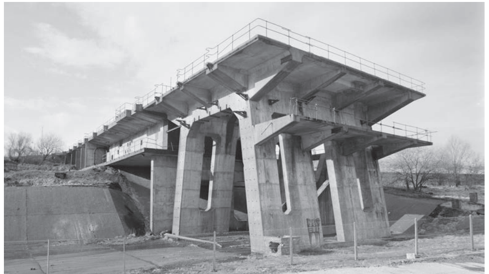
Fig. 16 Spadeadam, Cumbria, Greymare Hill, C2 test stand, when the Blue Streak missile was cancelled in April 1960 this stand was left unfinished, scheduled. (© Historic England AA94/2010)
