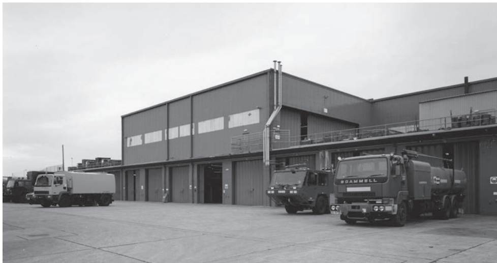
Fig. 24 RAF Wittering, Peterborough UA, purpose-built Blue Steel storage facility with garages for AEC Mandator missile transporters, Listed Grade II. (© Historic England AA99/09838)
