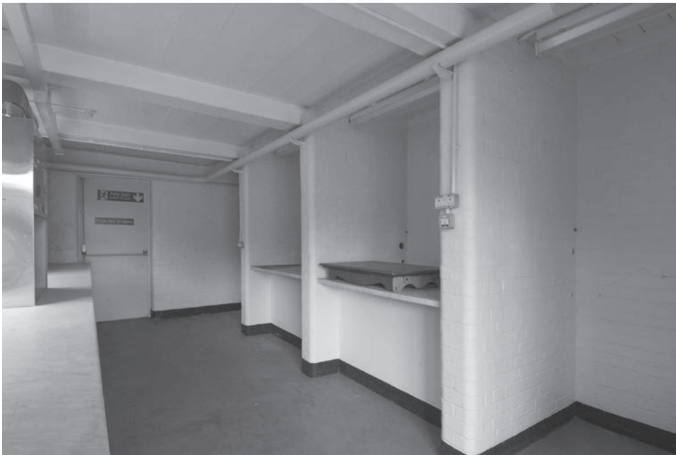
Fig. 2 Fort Halstead, Kent, Experimental filling shed F11, interior showing the vertical filling bays. (© Historic England DP060548)
