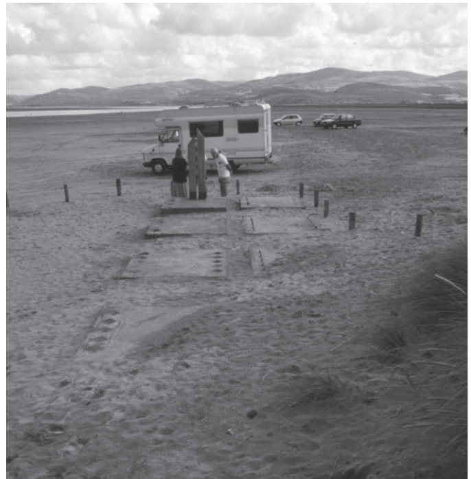
Fig. 4 Ynnyslas, Dyfed, the footings of the launch rail for the LOGGAP test bed. (© Wayne D Cocroft)
