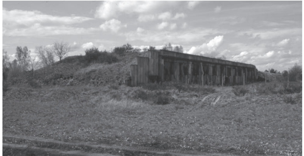
Fig. 38 Altengrabow, Germany, 1980s Soviet missile store, common practice in the Soviet armed forces was for warheads and missiles to be stored separately under the control of different units. (© Wayne D Cocroft)
