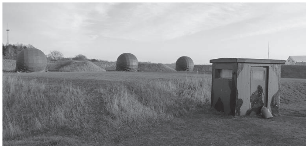
Fig. 36 Stevns Fort, Denmark, a 1980s Hawk missile battery with its radars protected by weather covers. (© Wayne D Cocroft)
