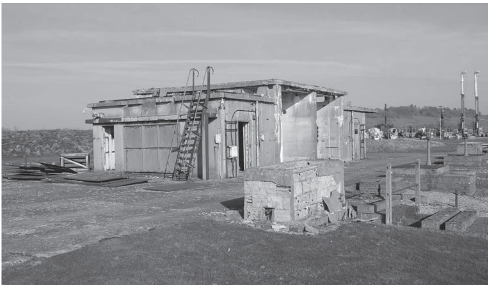
Fig. 7 Westcott, Buckinghamshire, rear of test stand C showing the oxidant and fuel bays, entrances to the monitoring rooms, and drains for removing unspent fuel and cooling water, Listed Grade II. (© Wayne D Cocroft)
