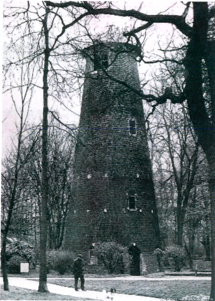
The Tower showing a double row of port holes which supported the reefing galley for the sails.
