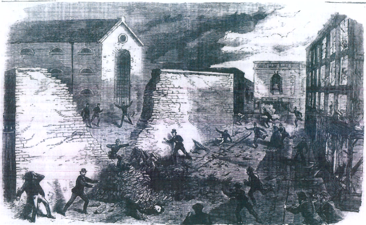
HOUSE OF DETENTION, CLERKENWELL—SCENE AFTER THE EXPLOSION.
