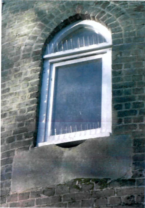
The shaped stone lintel under the second level window
