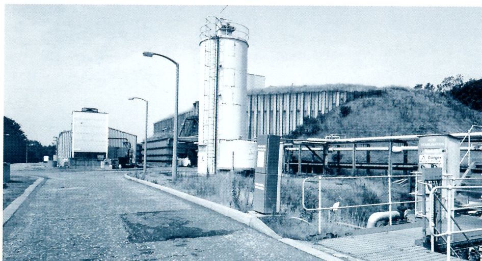
Plate 41: Exterior view of PETN Plant, 1995 (RCAHMS, C60223)
