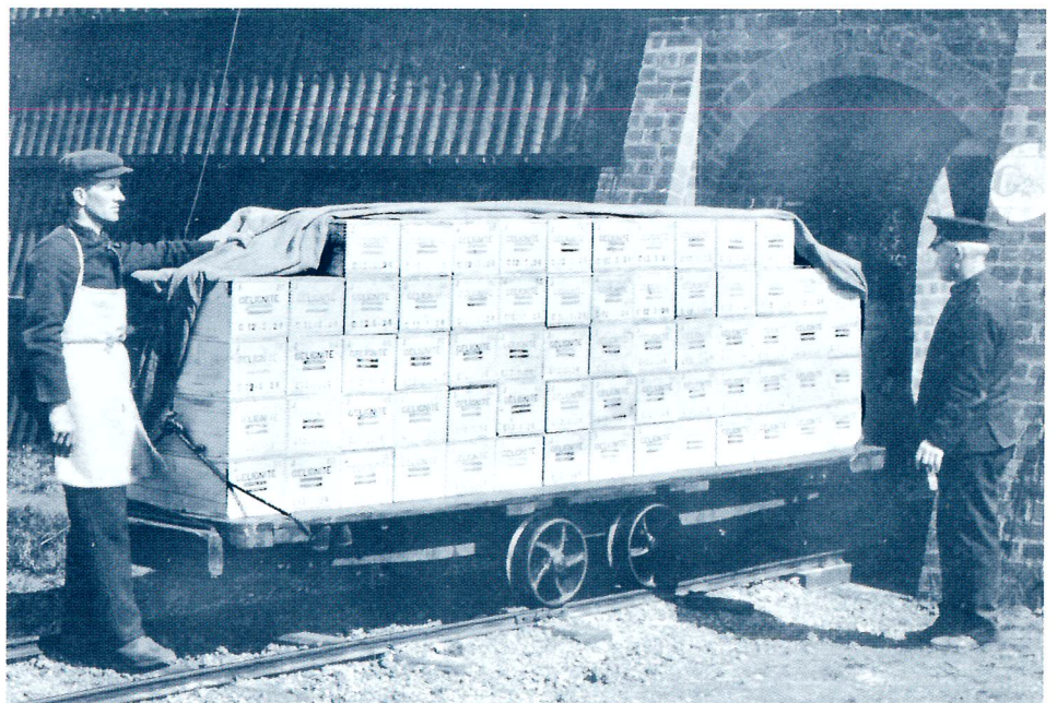
Plate 46: Blasting Department: view of bogey with finished cases of Gelignite leaving a packing house on the narrow gauge railway, and being taken for storage in a Magazine. The view also illustrates the steel-re-inforced mounds surrounding these and other types of building in the Danger Areas, circa 1925 (ICI Explosives, C65514)
