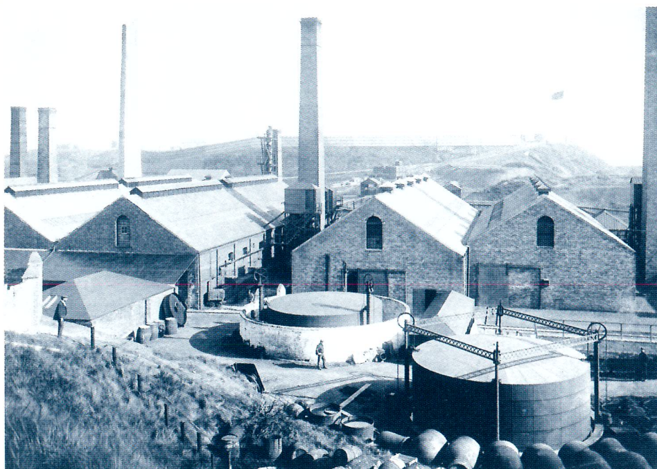
Plate 5: View within Ardeer Factory of nitric acid plant, with nitro-glycerine hill to right in background, and gas works in foreground, circa 1880. (ICI Explosives, C62977)
