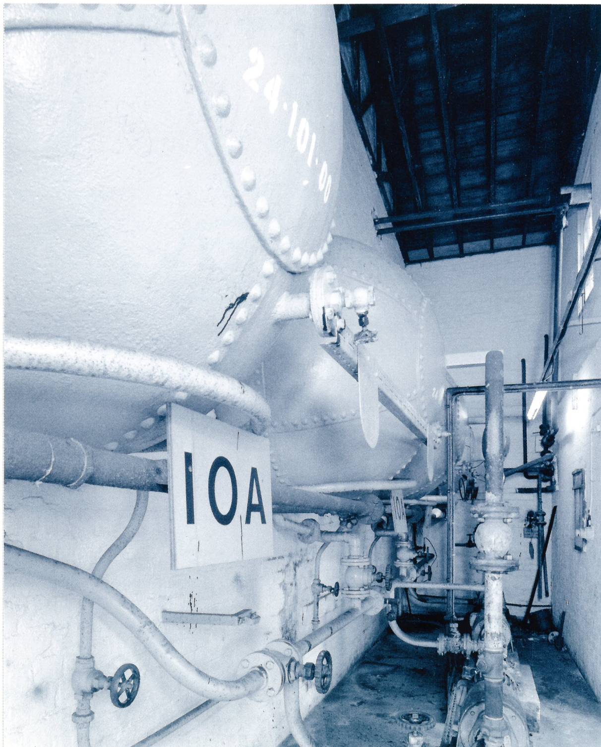
Plate 56: View of dome-ended former egg-end boilers, used to store glycerine and glycol at the foot of Nitro-glycerine Hill No.2, 1995 (RCAHMS, C60076)
