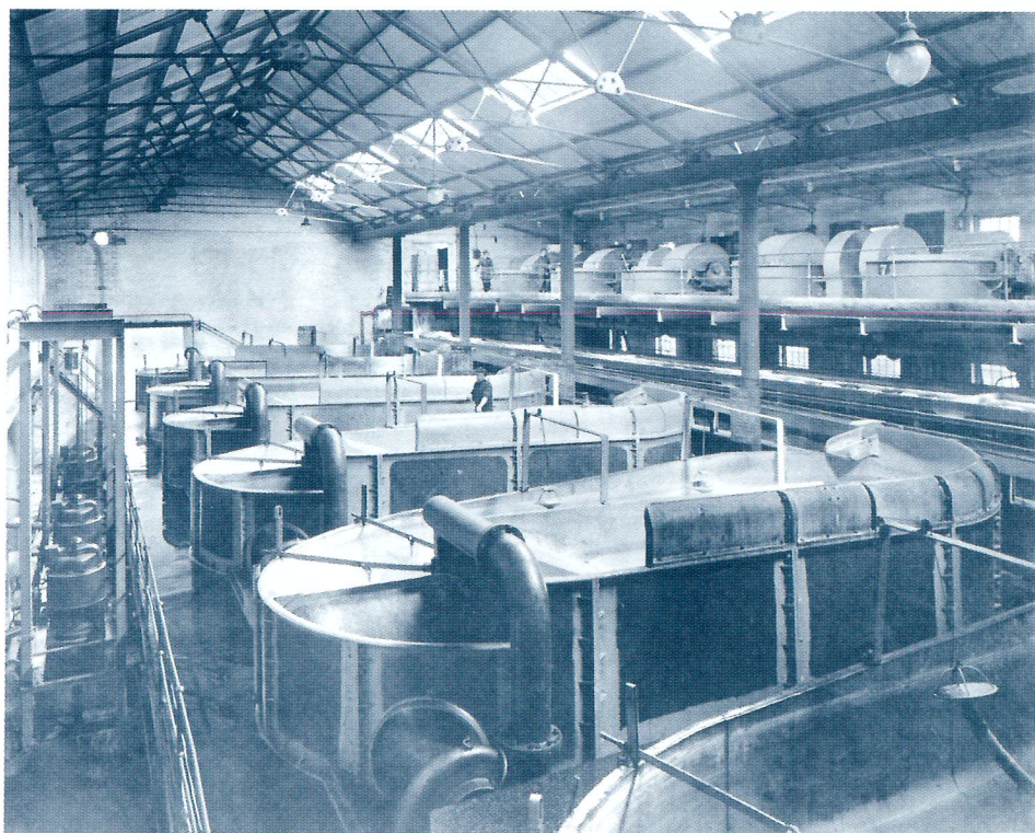
Plate 32: Interior view of Nitro-cotton pulping and finishing house showing potchers and pulpers, circa 1925 (ICI Explosives, C65320)
