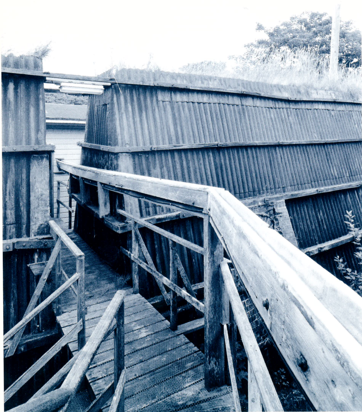
Plate 57: View of AC2, a 'C' House on Nitro-glycerine Hill No.2, showing the wooden gangway and lead-lined gutter approaching through a gap in the Chilworth Mound, which isolates the building, 1995 (RCAHMS, C60084)
