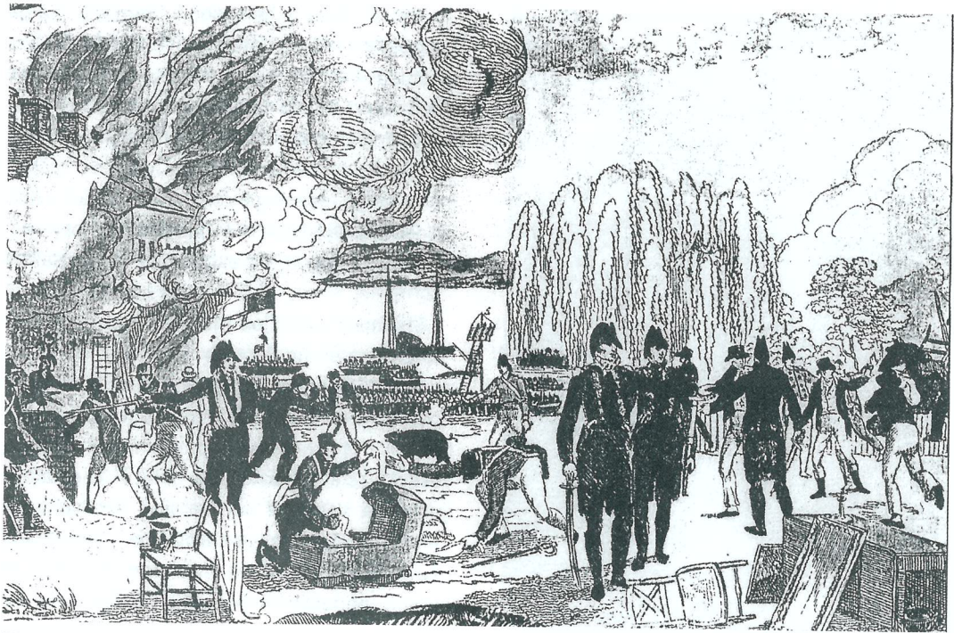
Fig. 9 A rare scene that includes a British rocket equipment in action during the War of 1812, the action at Havre de Grace, Maryland, on 1 June 1813. Note that Fig. No. 5 in this scene is called a "Machine for throwing rockets" in the original colour etching. It is seen as a ladder-like frame launcher and was adjustable for launching at different angles. Fig. No. 2 is 1st Lt. George A. Westphal who, although suffering from a previous wound (note the arm sling), had commanded some of the rocket boats used in this assault, although not shown with the rockets. (Original etching in the Maryland Historical Society)
