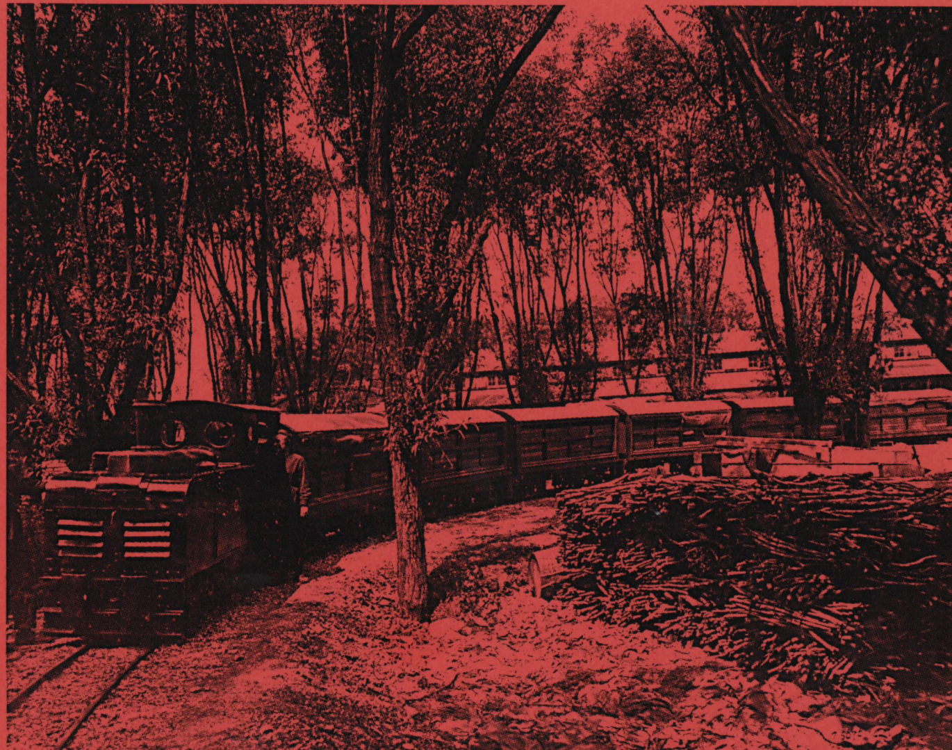
ZLH locomotive in the woods on the North Site of the Gunpowder Factory with a rake of six cordite wagons. Note in the right foreground a large pile of cut Alder wood, which is indigenous to the site, drying in preparation for conversion to charcoal. (RARDE)
