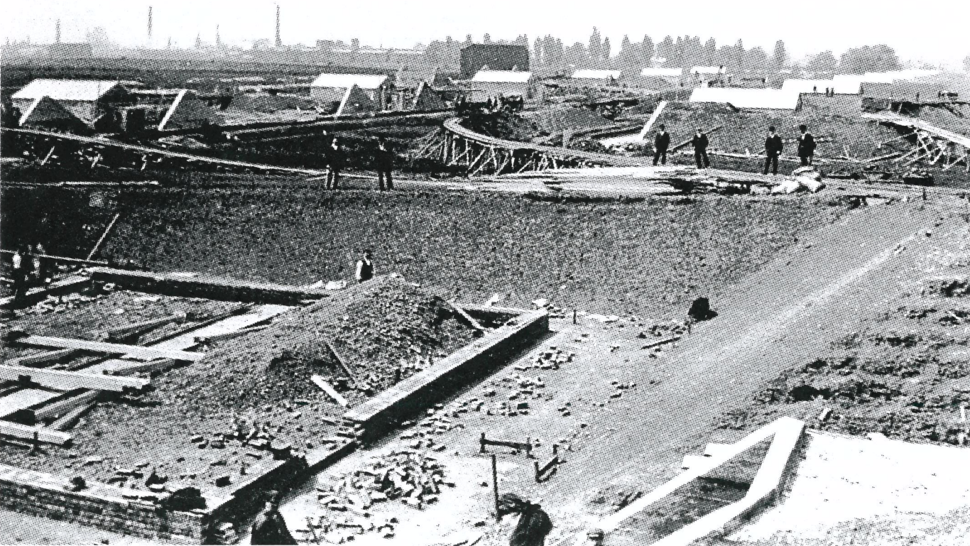
The two photographs above show the construction of the South site cordite stove complex, with horse drawn tipping wagons in use. (RARDE)
