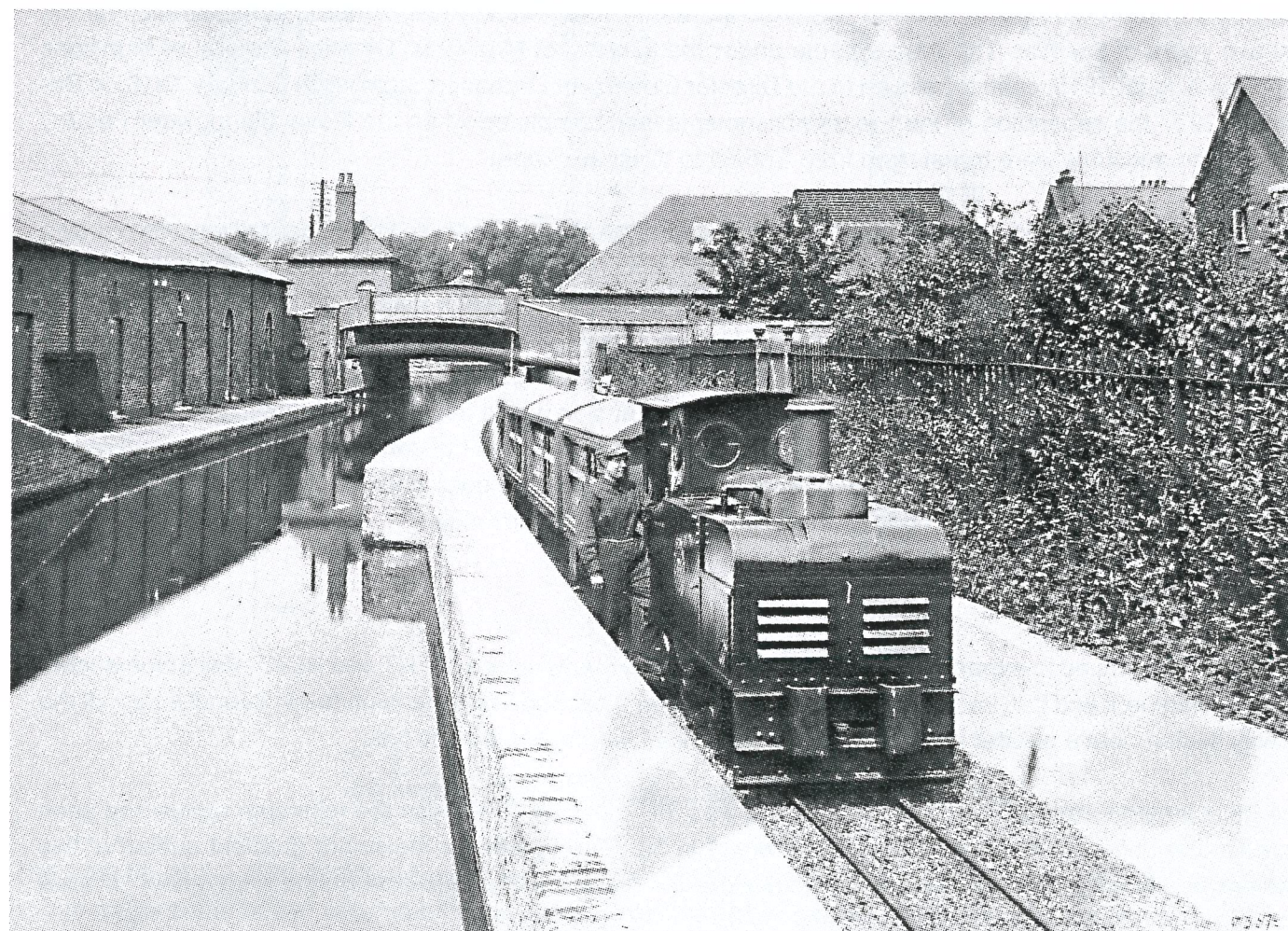
Ruston Proctor ZLH with a train of three wagons exit the Highbridge Road Tunnel. (RARDE)
