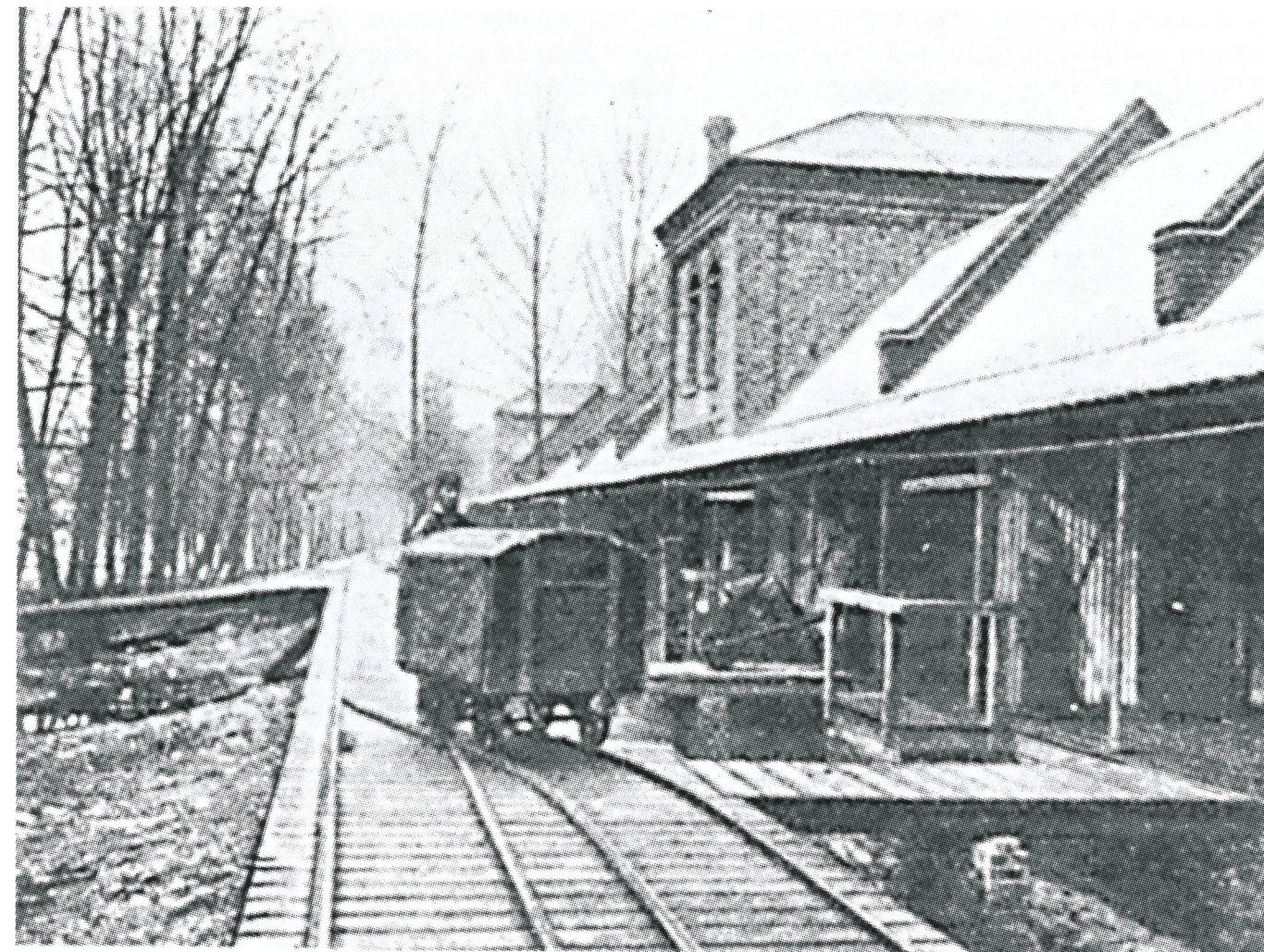
This photograph, which appeared in the Strand Magazine in 1895, gives a good impression of the wooden track and hand-propelled wagons in use at that time. The gauge of the track is thought to have been 2ft 3in.
