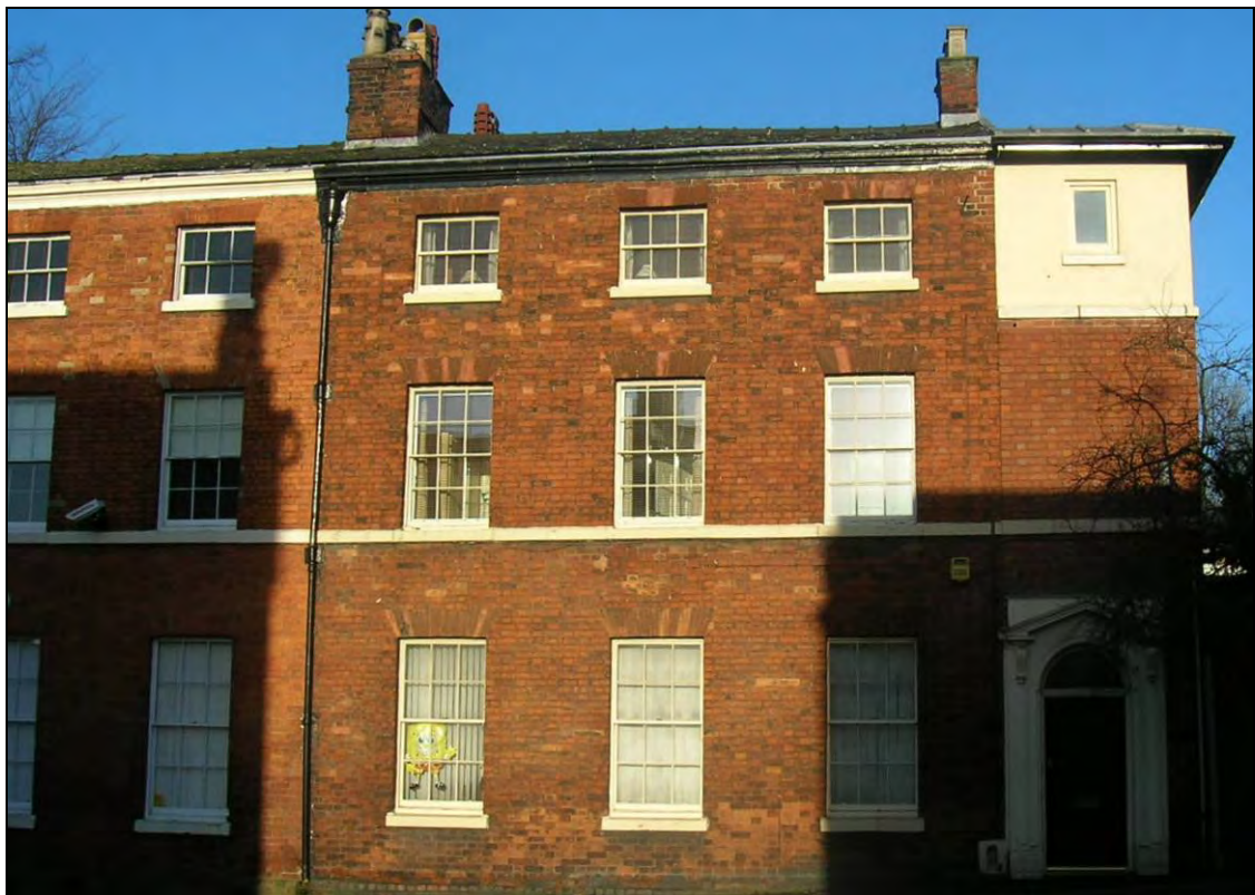
Figure 20: SRN: 5050 – Grove House in King Street, Newcastle-under-Lyme, registered as a War Supply Depot in 1915
