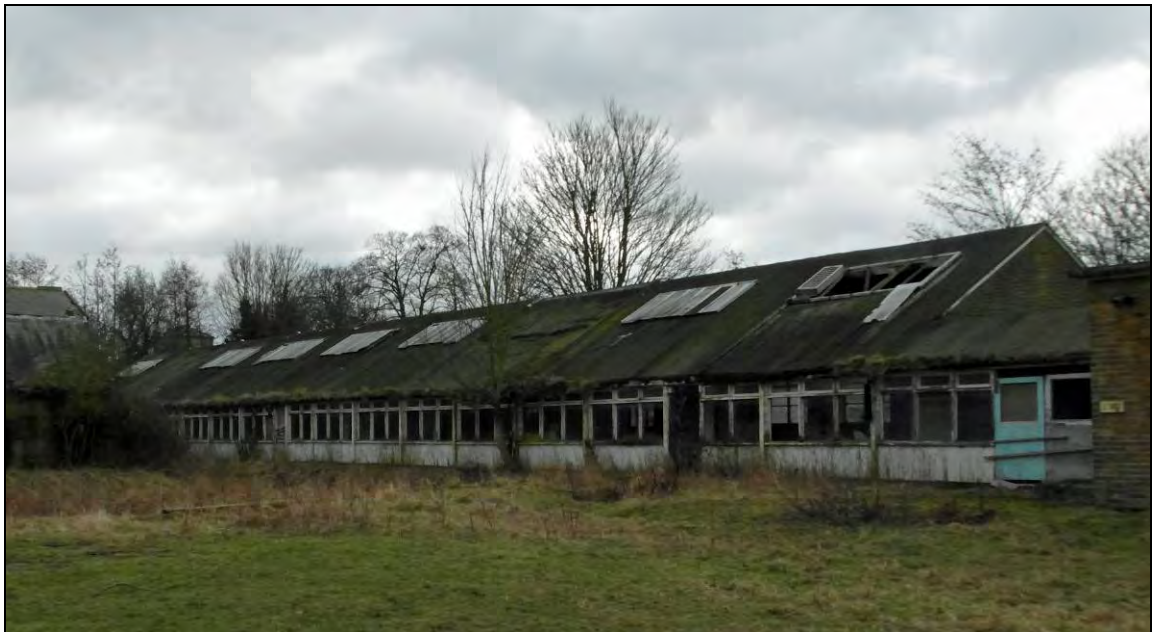
Figure 27: SRN: 502 – Present condition of Cordite Press House No. 5, Royal Gunpowder Mills
