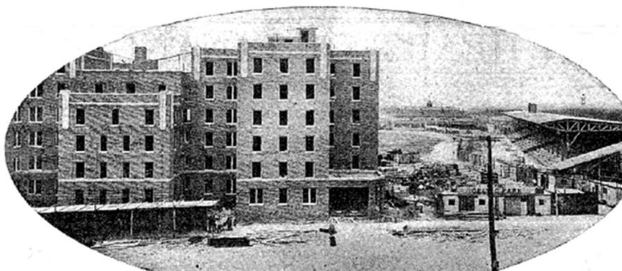
A photograph in The New York Times real estate section in July 1931 shows construction of the Celtic Park apartments, before the demolition of the old grandstand (right) and pavilion (distance). The ticket gate with the Celtic Park marquee can be seen in the bottom right. This photo was taken from the corner of 43rd Street and 48th Avenue, looking south.
