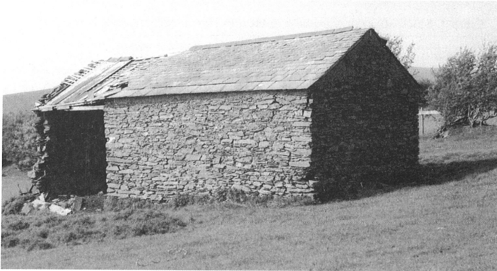
FIG. 9. Photograph of the building considered to have been the former Poaka Magazine on Lindal Moor, from the south-east. (Photograph by Dave Robson.)
