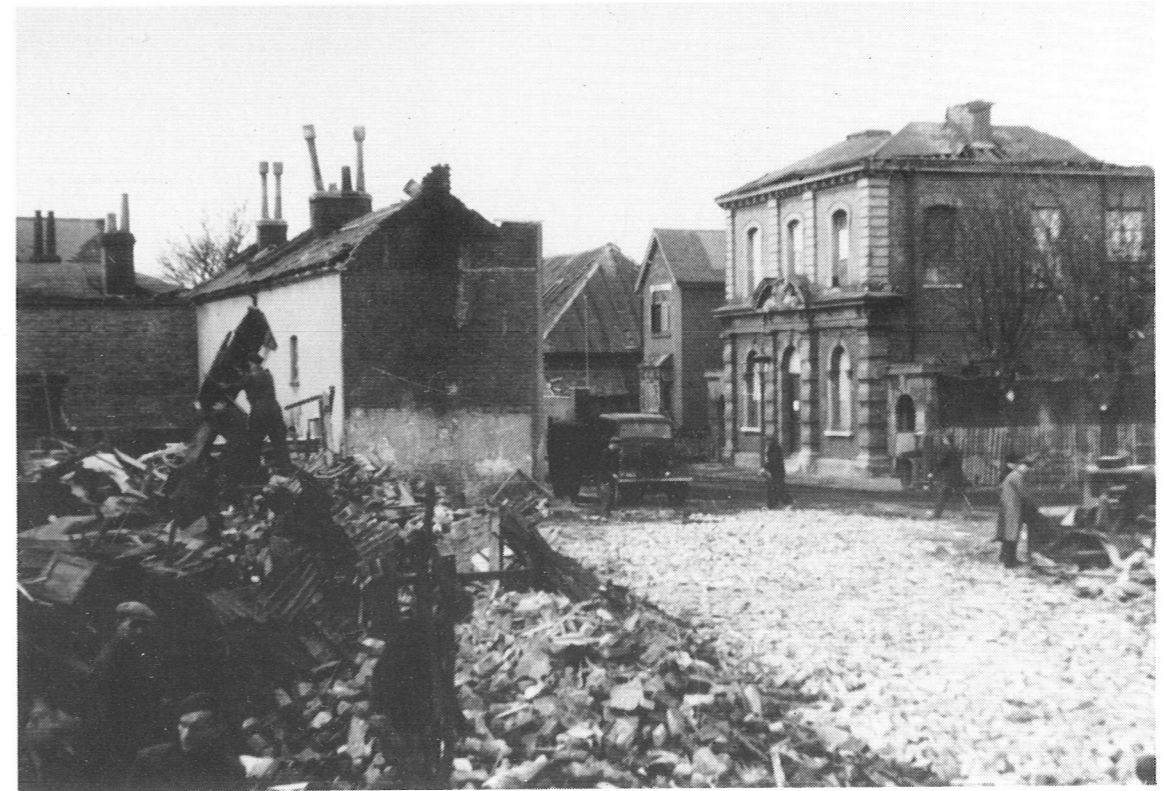
Highbridge Street - temporary roadway page 43
