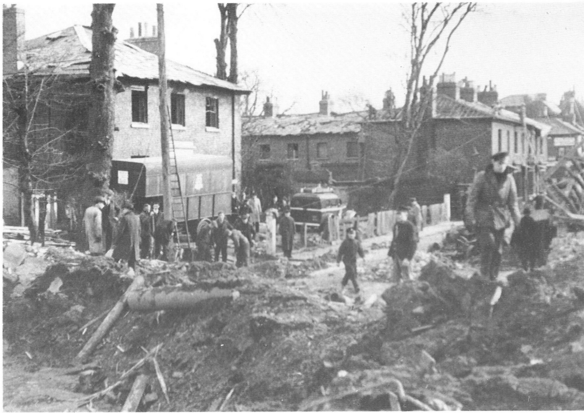
Highbridge Street - emergency repairs page 42
