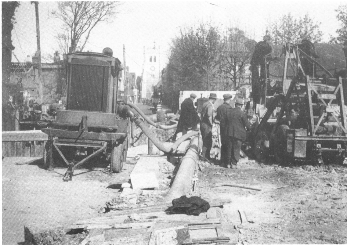
Highbridge Street - heavy machinery in use page 43
