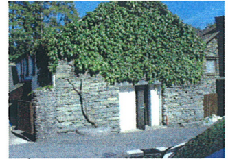
The mixing or preparing house. The column at the left was part of the wheel pit where a waterwheel would have been used to drive the mixing process.
