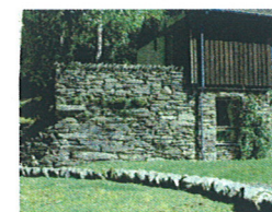
Surviving fabric at the West end of mill 5, rebuilt when Lodge 16 was erected.
