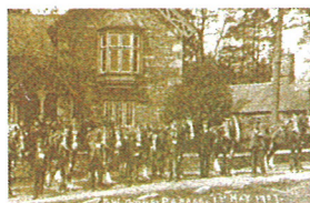
Beech Tree House - where the hoopers and coopers made the barrels for shipping gunpowder.
