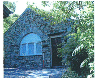
Southern gable of the saltpetre store showing the blocked cart entrance.
