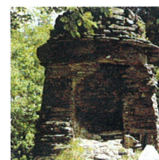
Chimney for the Stove House by the Country Club.
