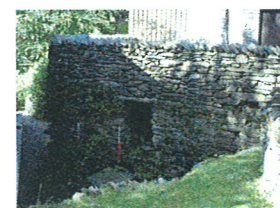
Remnants of Mill 6.
