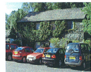
This photo of the Becks side bedrooms was taken before Becks side timeshare was built...it was the box-makers' house and the joinery. When the timeshare was built, the old stones were maintained and you can see the lintel and corner stones that were replaced.
