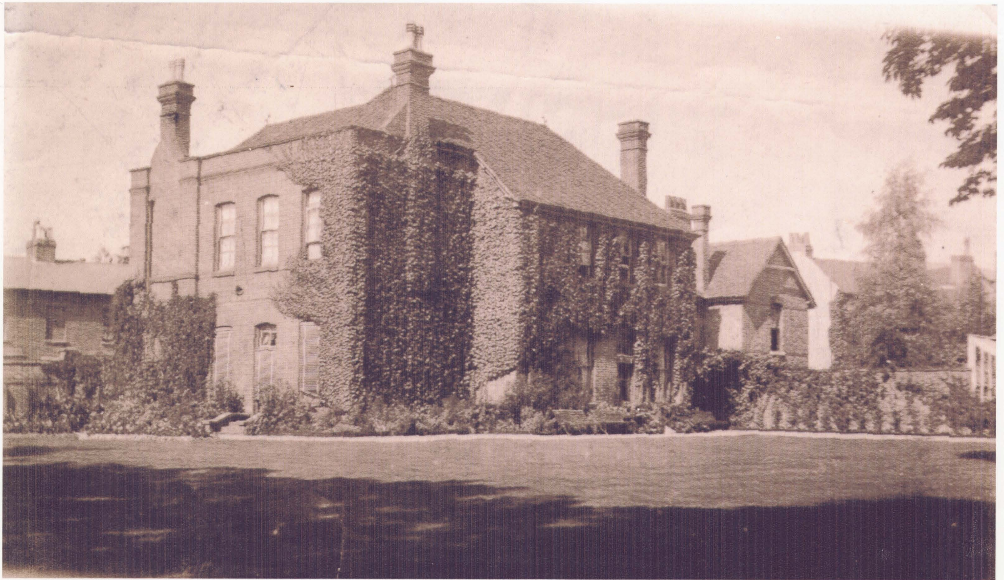
The Superintendent's House, The Royal Gunpowder Factory, Waltham Abbey. 'Government House', Highbridge Street. The Knapman's lived here from 1939 to 1950. (Mr. Knapman worked at the MoD (then the War Department?) from 1943 to 1950)
