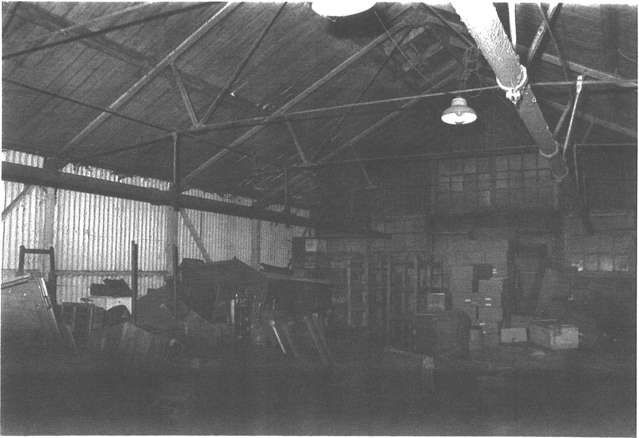
M349 PLATE 16 - GENERAL VIEW OF INTERIOR, FROM EAST DOOR
