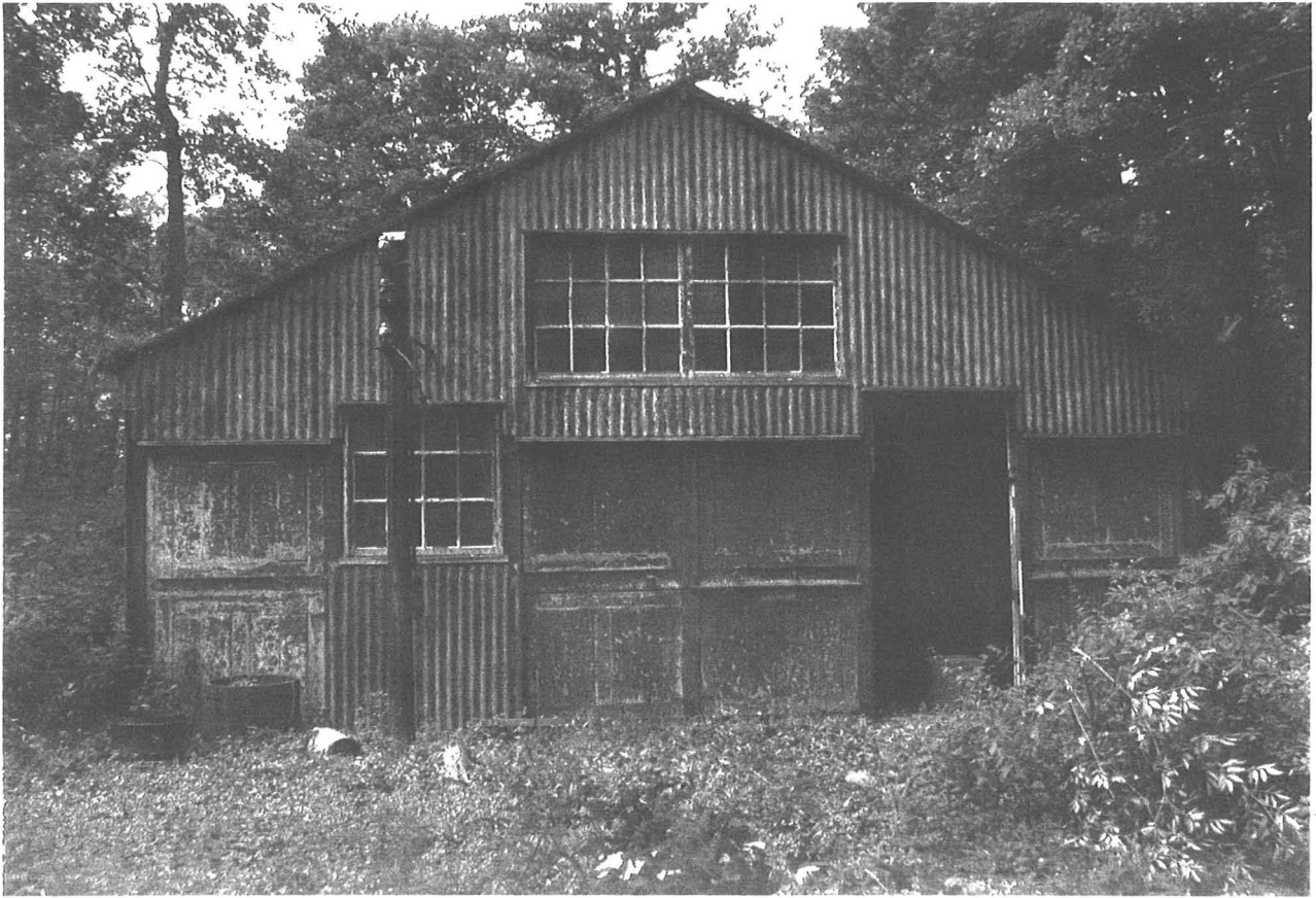
M349 PLATE 7 - EAST OF BUILDING, FROM EAST
