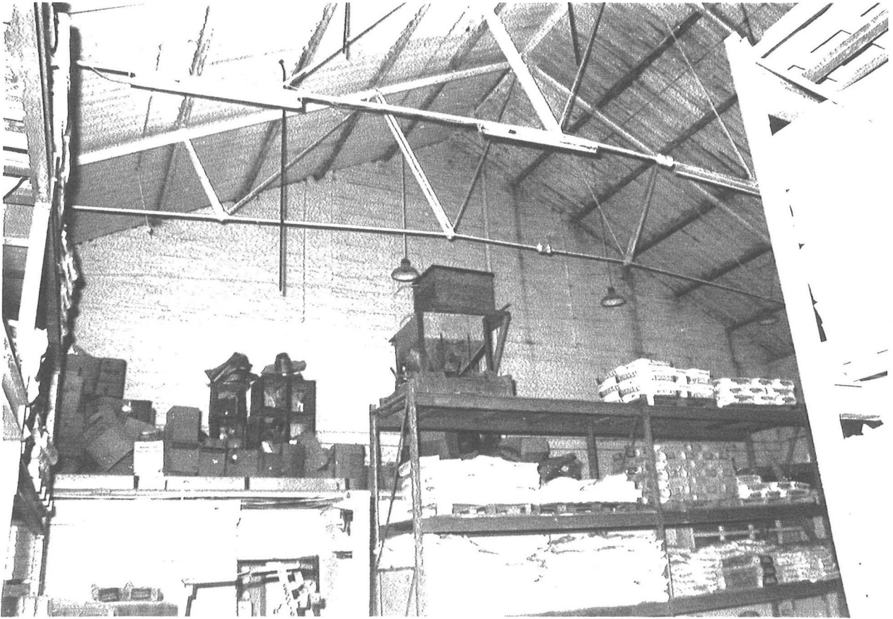
G431 PLATE 25 - DRYING ROOM, DETAIL OF WEST WALL AND ROOF
