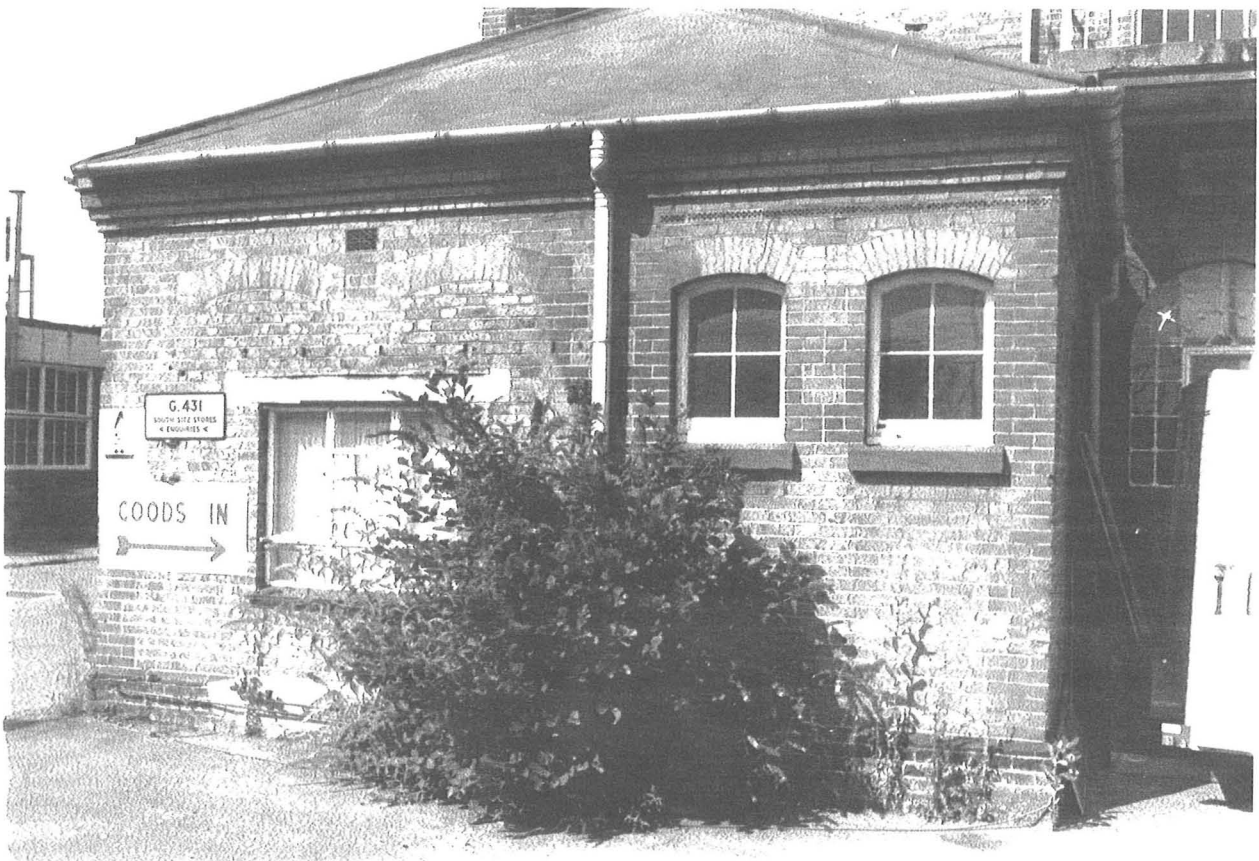
G431 PLATE 37 - EAST ELEVATION, EAST ANNEXE, FROM EAST
