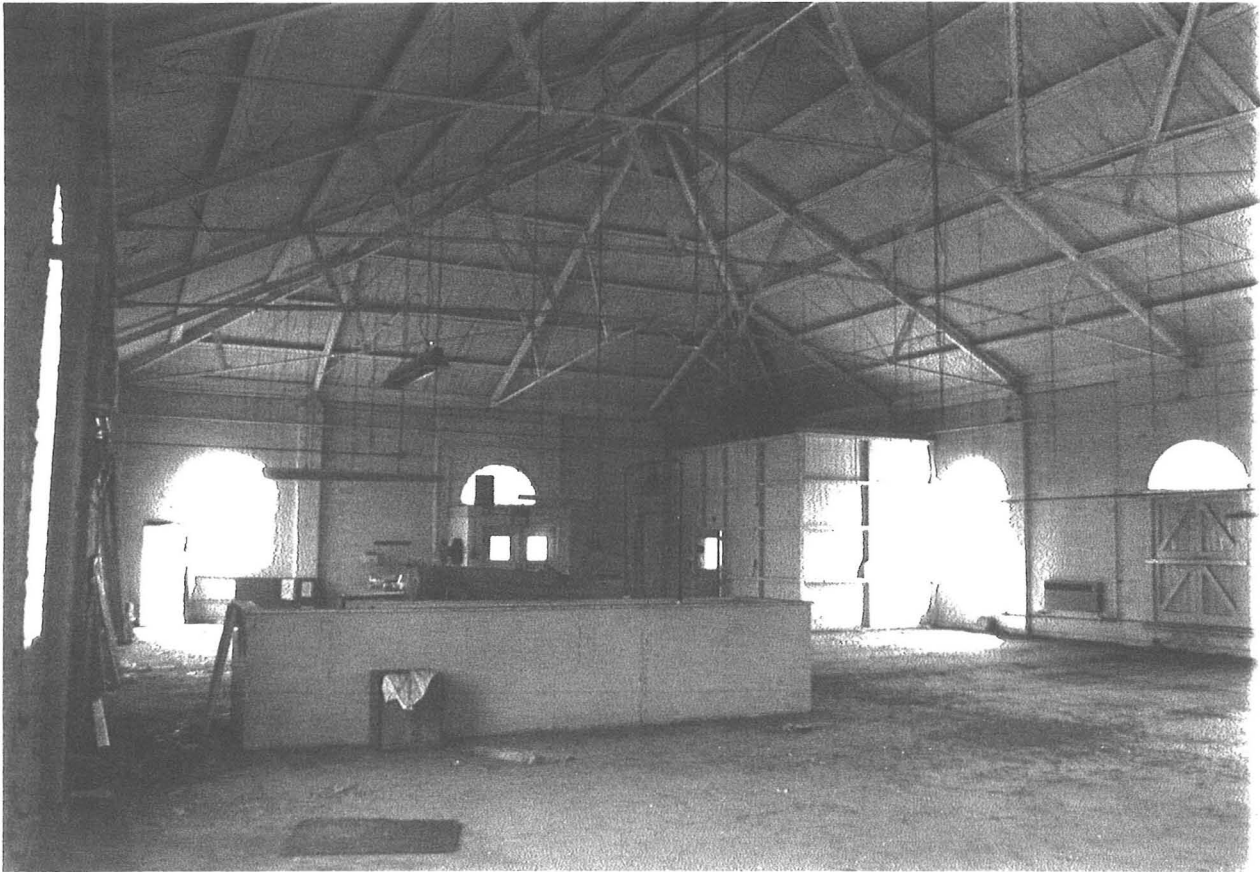
G431 PLATE 32 - FIRST FLOOR INTERIOR, FROM NORTH WEST CORNER
