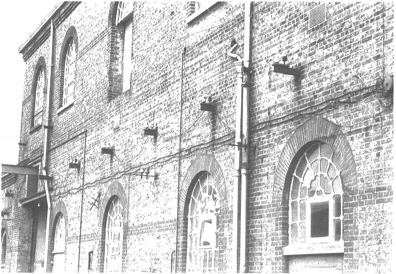
G431 PLATE 36 - CABLE/TELEGRAPH RUNS, SOUTH ELEVATION
