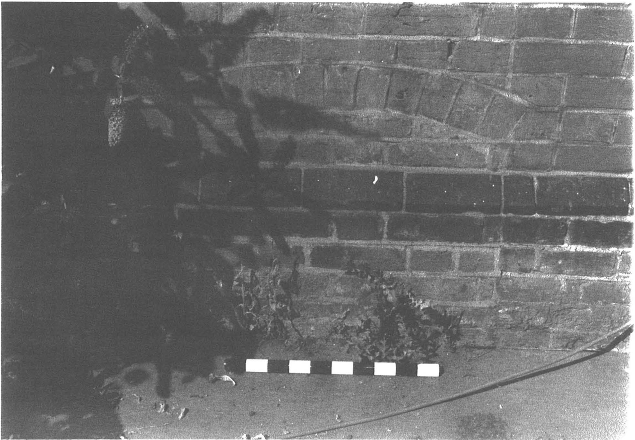
G431 PLATE 16 - BRICKED-UP ARCHED OPENING, EAST WALL OF EAST ANNEXE
