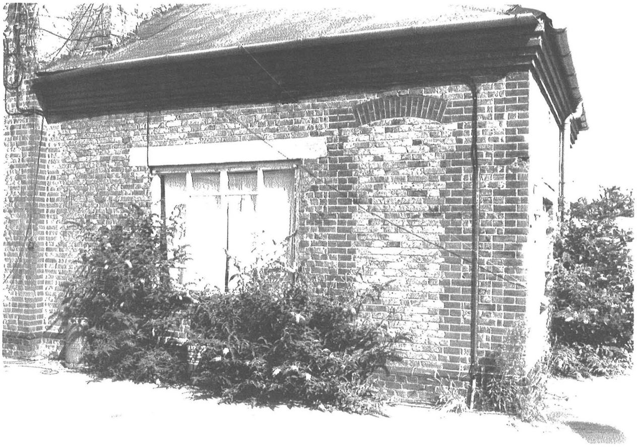
G431 PLATE 13 - SOUTH ELEVATION, FROM SOUTH
