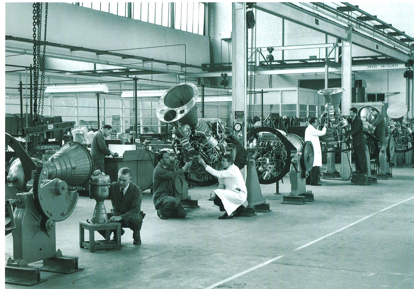
Figure 2.17 Stentor rocket engine production line at the Bristol Siddeley Ansty site, c. 1960. Over 120 Stentor engines were built: at the peak of production, an average of almost four were produced each week. (Rolls-Royce plc)
