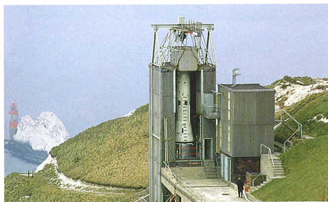
Figures 3.12 and 3.13 Westland Aircraft's Black Arrow test site at West High Down, Isle of Wight, c. 1969. Work on excavating the site started in 1956, shortly after the Saunders Roe company had been awarded the contract to develop Black Knight. The Black Arrow R0 vehicle is being readied (left) for test firing (right), where clouds of steam are clearly visible as thousands of litres of dousing water are vaporised by the heat of the engine's exhaust. (GKN Aerospace)
