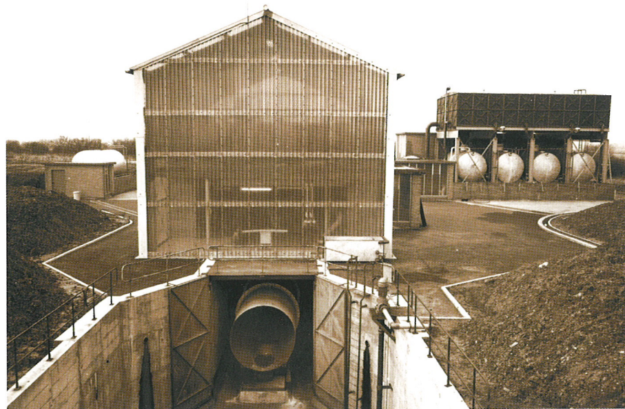
Figure 3.15 Gamma Type 8 engine static test building at the Bristol Siddeley Engines site at Ansty, Warwickshire, c. 1968. The opening of the exhaust duct can be seen beneath the building. (Rolls-Royce plc)
