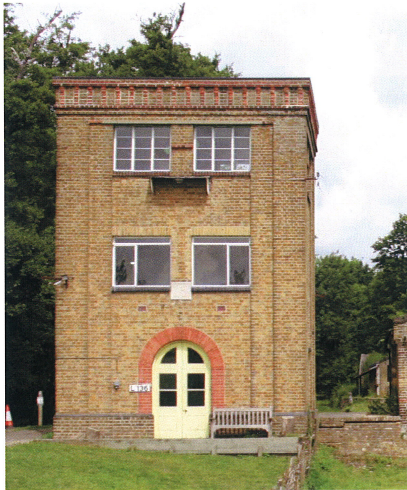
The Remote Accumulator Tower
