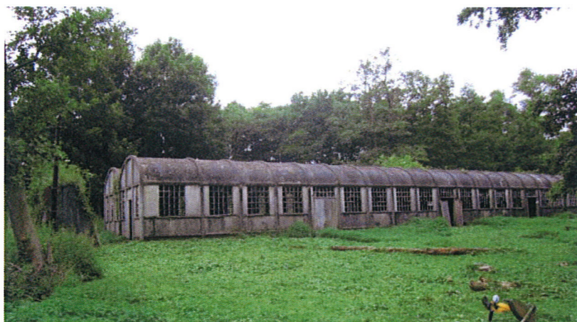
The Quinan Stove and one of its traverses (left)
