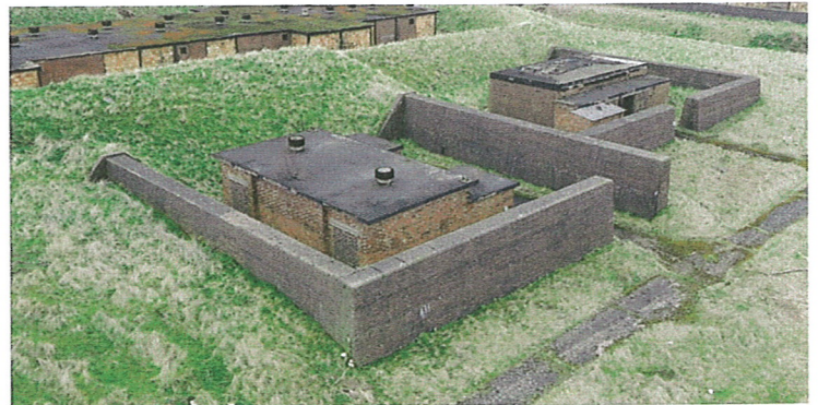
Right: Group 8 buildings constructed within blast walls and earthen banking
