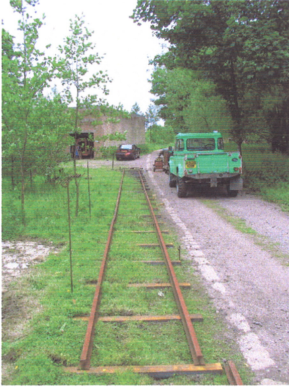
Track being laid in June.
