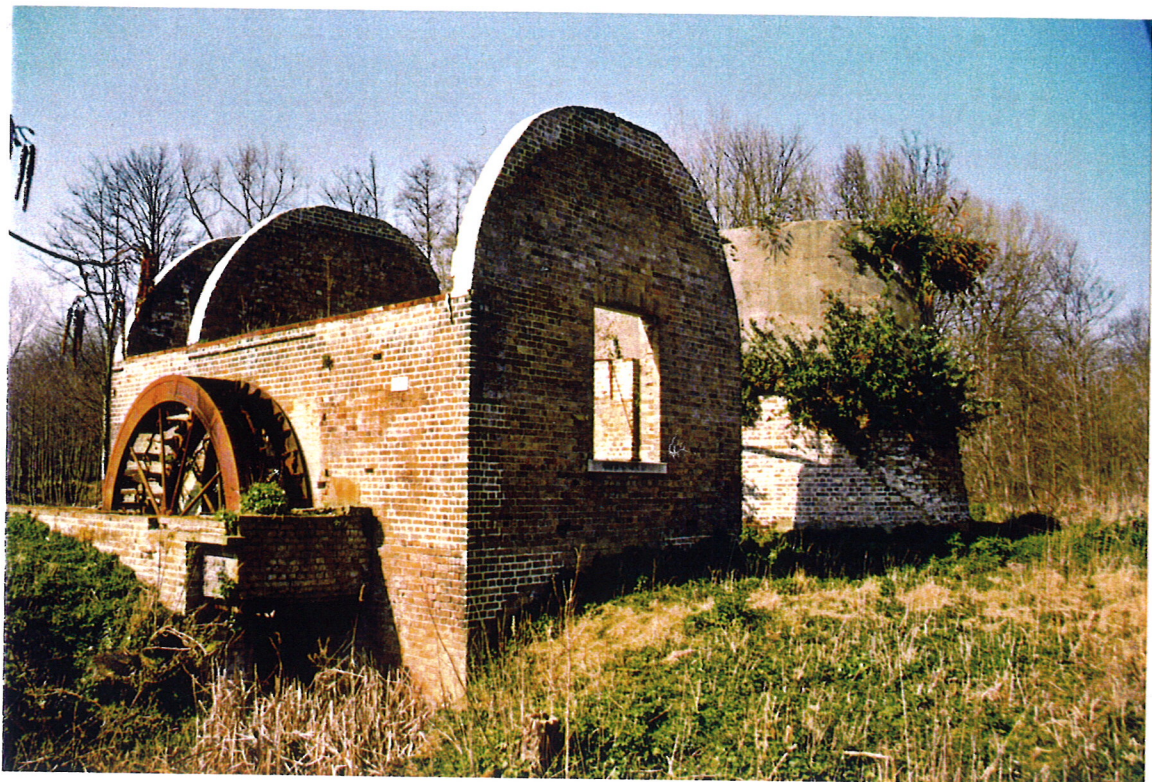
The waterwheel and pumphouse with the traverse beyond. The Royal Gunpowder Mills Waltham Abbey.
