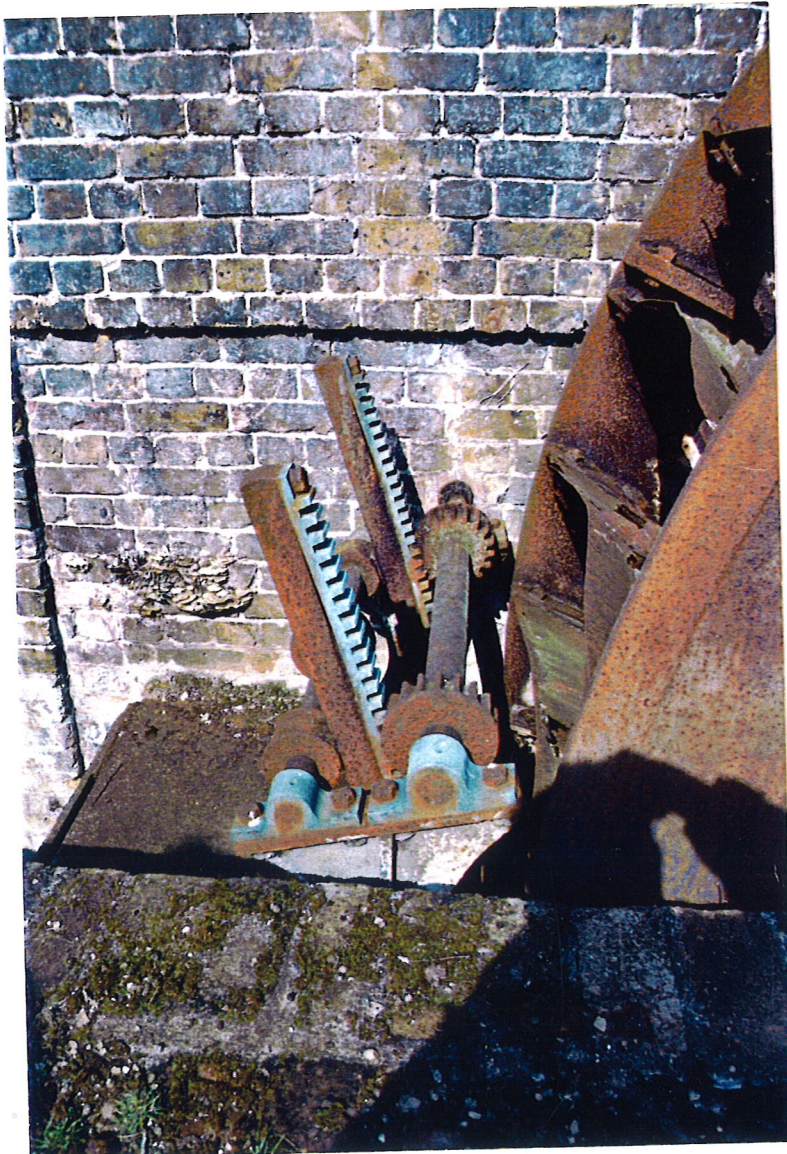
The inside of the pumphouse showing the linkage to the pumps from the waterwheel
