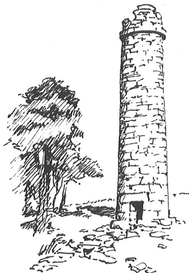
Figure 8. A chimney stack at Cherry Brook, Dartmoor (© R Oliver)
