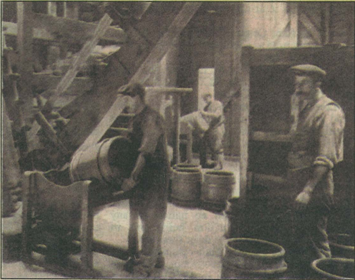
Production line: Men operating the Oare Gunpowder Works machinery, with its home-made barrels.
