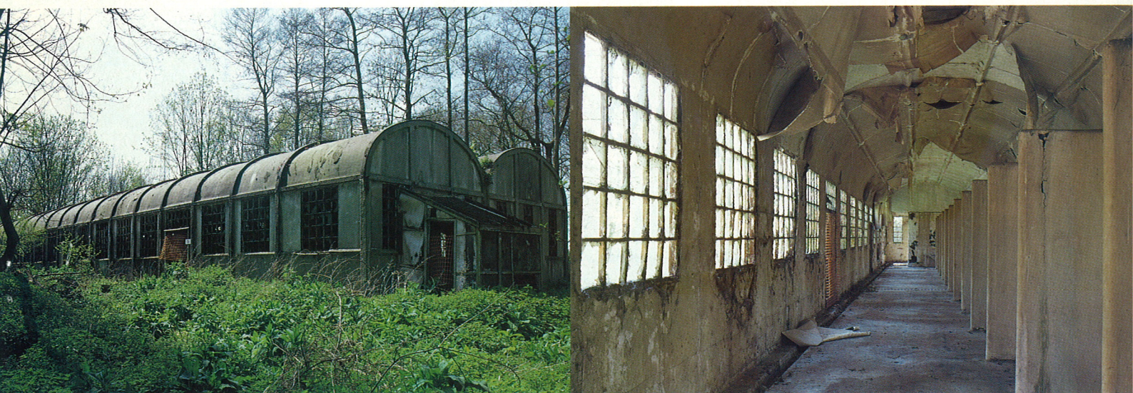
Above and above right: the Quinan Stove, 1936. Below: E-shaped concrete traverse beyond the Long Walk bend
