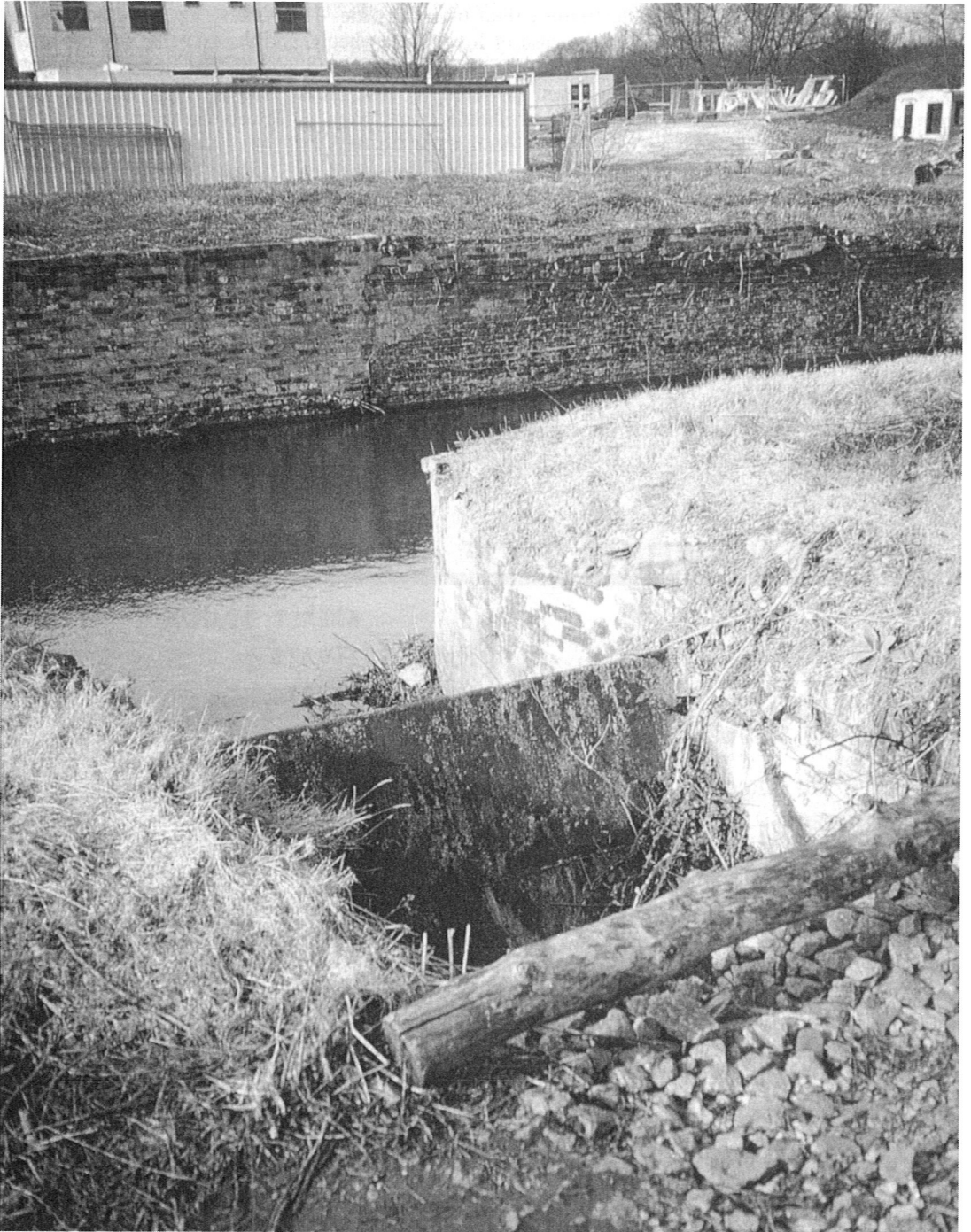
Fig. 13 The surviving iron 'crown of the fall' at the intake to Smeaton's Mill on the Millhead Stream at WARGM. Photograph by R. A. Buchanan.
