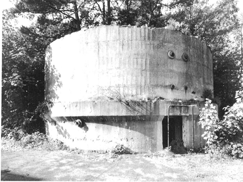
22 Figure 2. Royal Naval Cordite Factory, Holton Heath, Dorset, remains of the fermentation vessels used 23 for the production of acetone (BB94/16943) © Crown copyright.NMR
