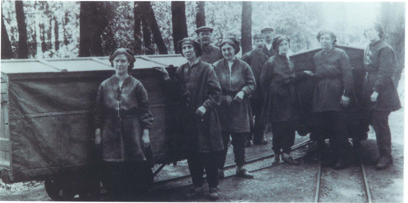
RGPF WALTHAM ABBEY. Hand propelled waggons with peaked roofs WW1. These smaller waggons were used within the process areas.
