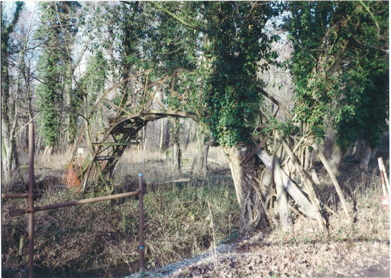
RGPF WALTHAM ABBEY. Footbridge over canal, built in 1878.
