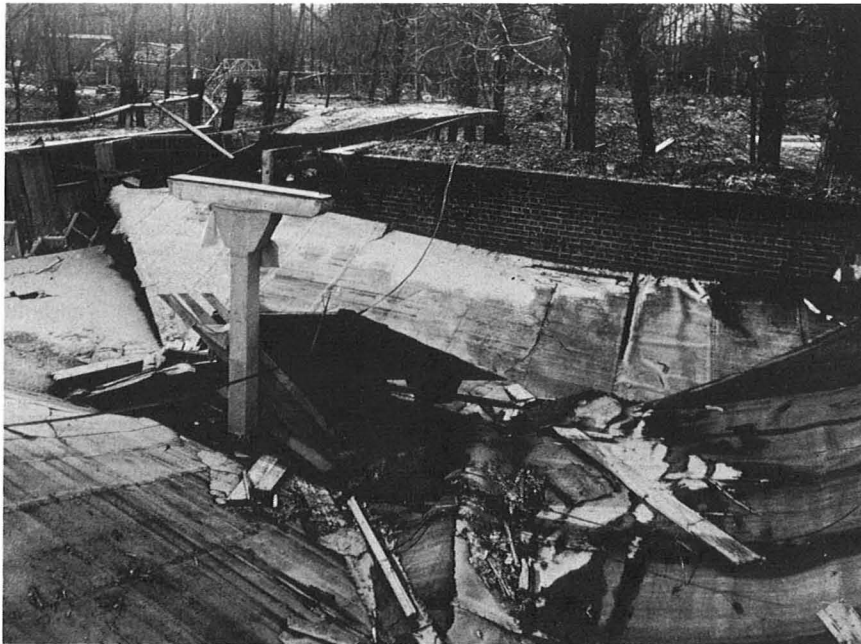
Left: No. 2 Weighing House after the first explosion looking south-west towards the Engine House alongside No. 14 Stove.
