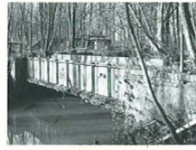
8 Cast-iron aqueduct, dated 1877-8
