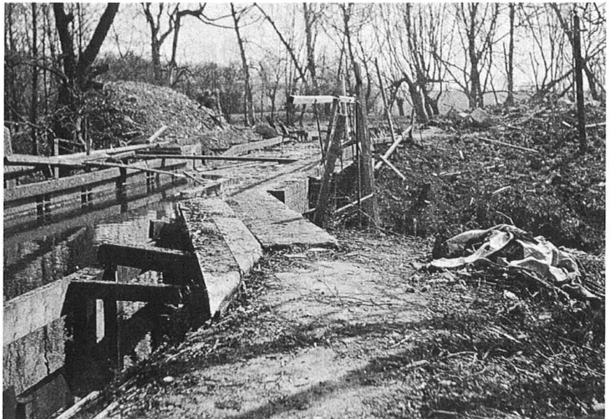
The pathway where Monk and Raby were killed was photographed for the record. At this point, an aqueduct (on the left) is carried in an iron trough over the waterway running below it at right-angles.
