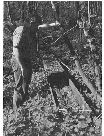
nitro-glycerine 'gutters' by which the explosive ran by gravity between buildings. Long since deprived of its lead lining, this particular one had a felt-covered wooden lid rather than the more usual canvas cover. It may be significant that this trough appears to have led towards the site of the ill-fated No. 5 Mixing House.
