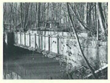
8 Cast-iron aqueduct, dated 1877-8
