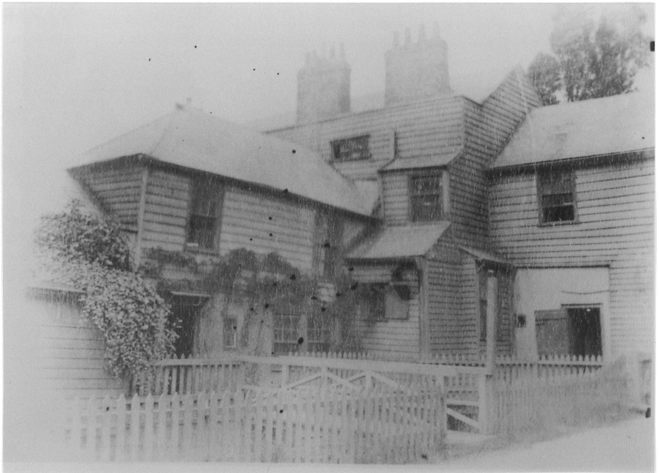
This wooden building, was the R.G.P.F. superintendent's, old quarters, south of Highbridge Street facing Powdermill Lane, with the old River Lea running underneath. Picture, 1885.
