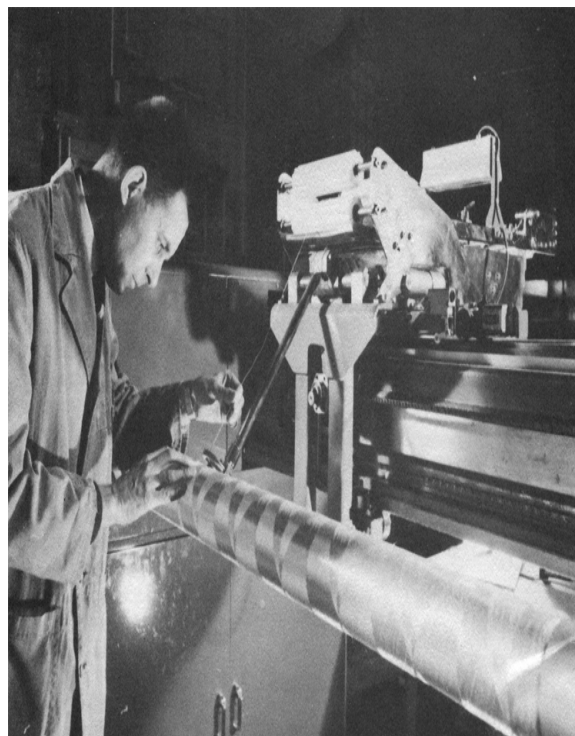
Fig. 10 Helical winding of rocket motor body.
