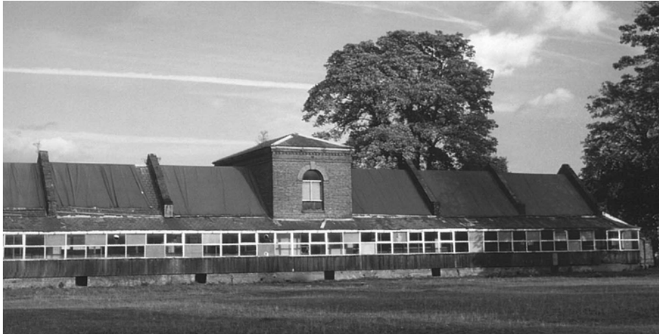
Fig. 1. Existing Steam Powered Incorporating Mill on North Site converted to Laboratories.
