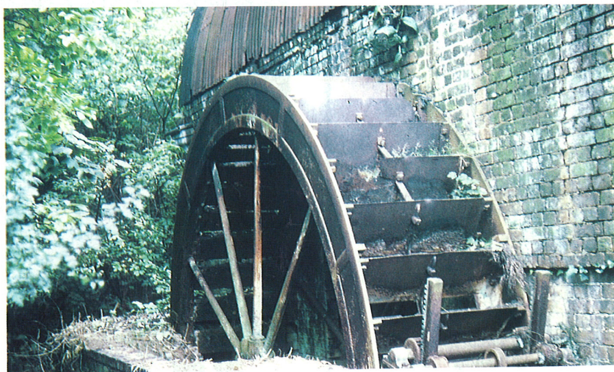
Water wheel for the Gunpowder Press House.
