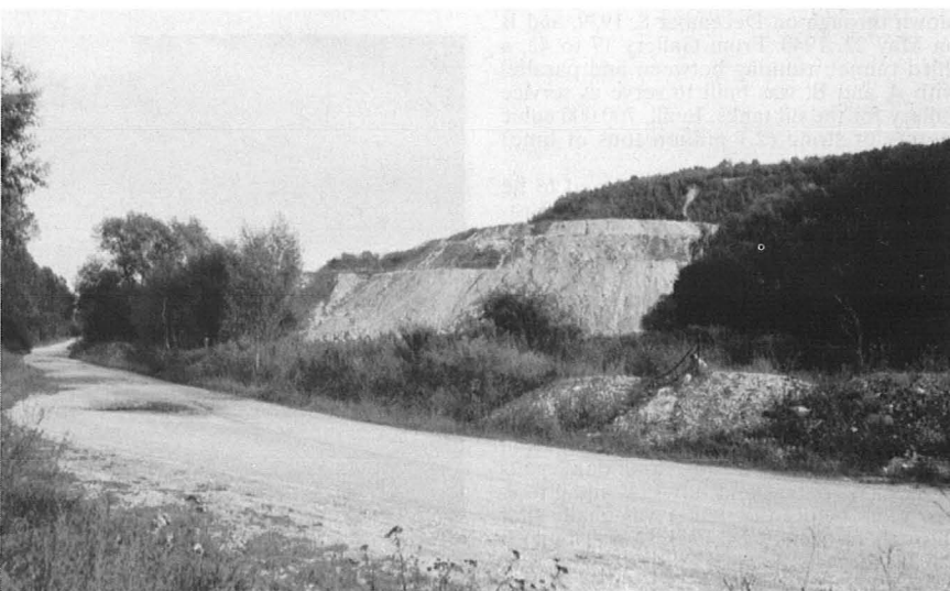
Today, both northern tunnel entrances have completely disappeared under a wall of waste stone dumped here by the Niedersachswerfen gypsum quarry.
