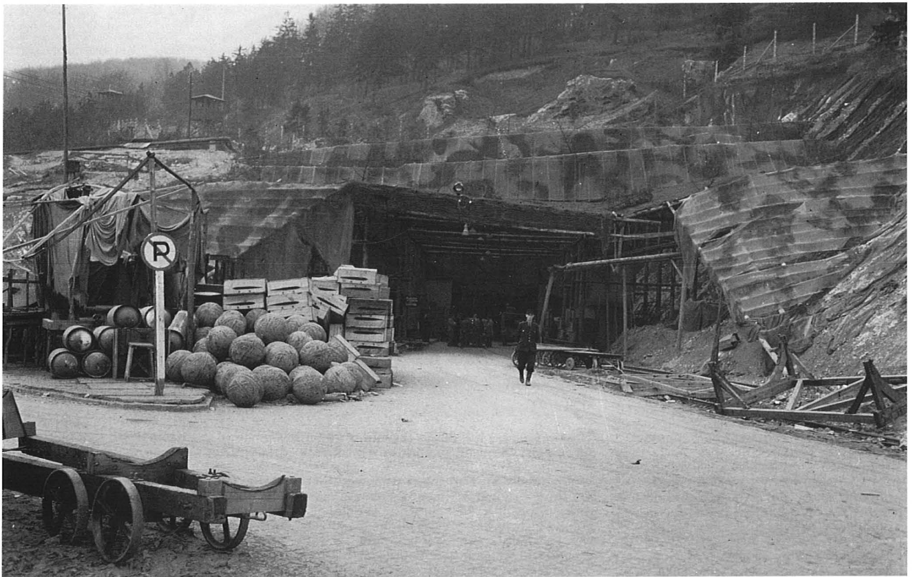
Although its southern entrance was already begun in 1941, Tunnel A was not finally opened all the way through until January 1944, the last 300 or so yards having been dug, under undescrivable misery and hardship and virtually with their bare hands, by concentration camp slaves. After August 1944,
