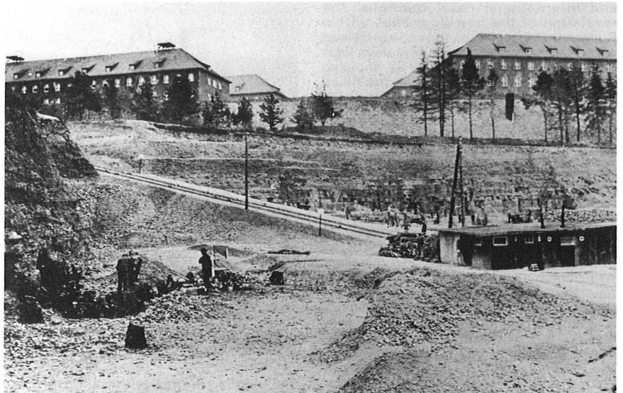
Air raid shelters for the use of the camp personnel were tunnelled into the side of the quarry which lay just west of the SS barracks. (BWA)
