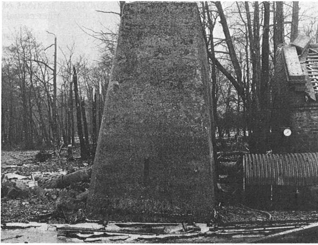
Left: Although this massive blast wall stood between No. 5 (about 250 feet away, out of the picture to the right) and No. 14 Stove, nevertheless the ton of gun-cotton in No. 14, which originally stood to the left of the wall, sympathetically detonated. However, although in direct line from the first blast, by some quirk the Engine House on the right still remained
