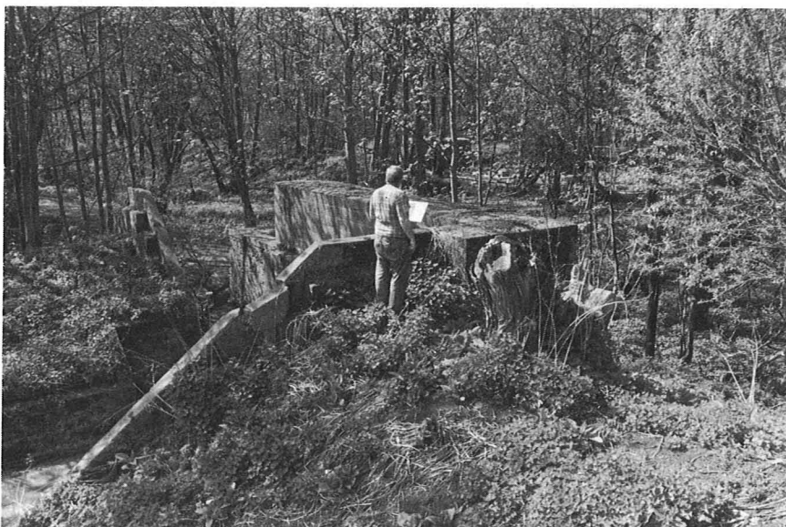
Having just been rebuilt, No. 2 Weighing House (Building 53A) was wrecked again in April so that the modern replacement (left), considerably enlarged and bearing a different building number (S27), bears little resemblance to the original. The footbridge is hidden in the trees. Right: An unexpected discovery in the nearby undergrowth was the remains of the old
