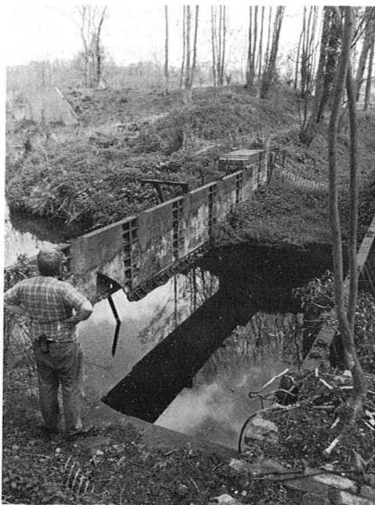
Left: The iron of the one-time aqueduct (Bridge 20) is now smashed and no longer carries water although the canal which runs below still feeds Newton's Pool. However, from the
