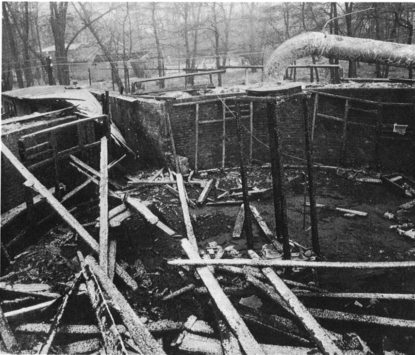
Just 200 feet to the south of No. 18 lay the old dry Stove No. 19. The wooden structure caught fire, this picture giving a good illustration of the method of constructing the inner building inside the protective mound. The view is looking west across the truck line, towards No. 14 Stove and the Engine House.
