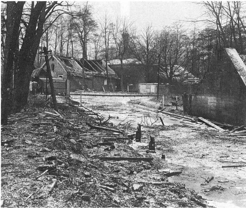
Another good comparison, although one which caused us a lot of head-scratching, was this one which we assumed was taken looking along a road towards one of the blasted buildings on North Site. The Court of Inquiry annotation stated that it showed the 'C.E. Magazine', fortunately also describing it as 'Building 89'. Although this did not appear on the associated drawing on page 37, reference to the plan produced for the Inquiry after the second large explosion on April 20 (page 36) did indicate its location.
