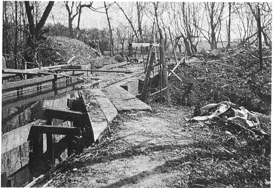
The pathway where Monk and Raby were killed was photographed for the record. At this point, an aqueduct (on the left) is carried in an iron trough over the waterway running below it at right-angles.
