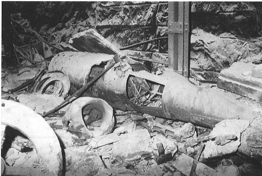
Heaps of V1 parts lying about in Gallery 45. As a result of the 1948 Soviet demolitions, many of the double floors collapsed, causing the parts stored there to spill out on the bottom floor.
