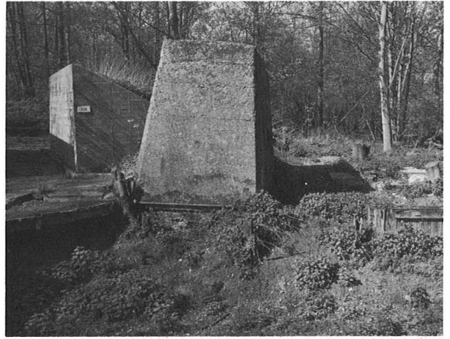
standing. The picture was taken looking due west from across the waterway. Right: For some reason, the upper section of the wall was later removed but the shuttering marks on the end clearly match up. The engine house has since been dismantled. In the foreground, the dry bed of the canal. The rough bridge on the left is a recent addition.
