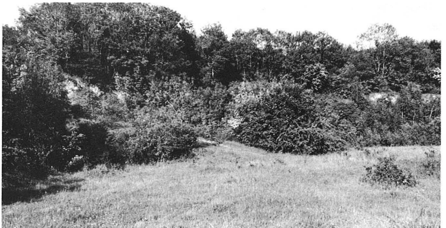
All but six of the SS barrack blocks were demolished in the 1950s. (See plan on page 2.) Of the rest, only foundations remain but the ramp of the tip-cart rail line from the quarry floor can still be discerned.
