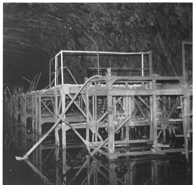
Left: At the end of the assembly line, the V2 would reach Gallery 41, where, by means of a mobile crane, it would be put upright for final testing. No. 41 was the only tunnel sufficiently high to encompass for the 14-metre (47-foot) missile, its extra-deepened floor giving it a ceiling height of 15 metres. Note the pools of ground water. Above: In the underground world of the Kohnstein today, only the top of the test stand sticks out of the water. Too deep in the mountain for us to be allowed to photograph it, this spectacular picture was taken especially for us by Alvin Gilens in March 1998.
