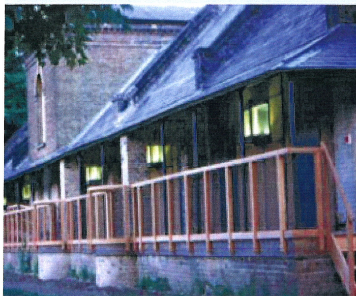
Steam powered incorporating mill.
