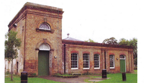
The engine house has been restored by volunteers.
