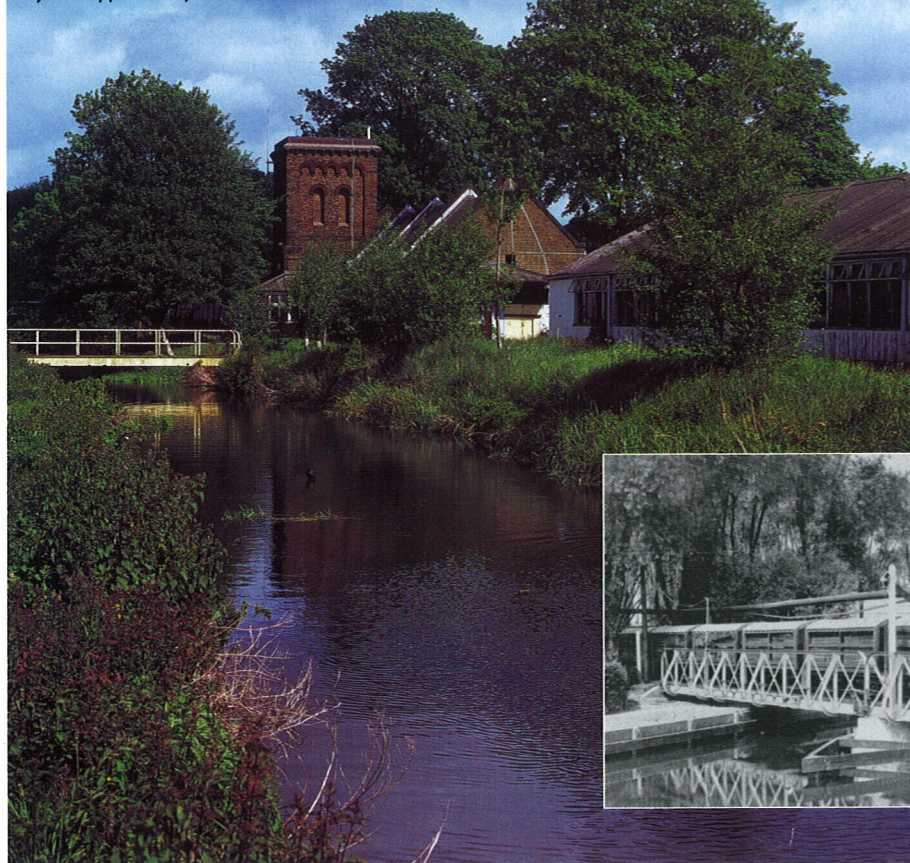
Some stretches of the former canal system appear ready for use.
