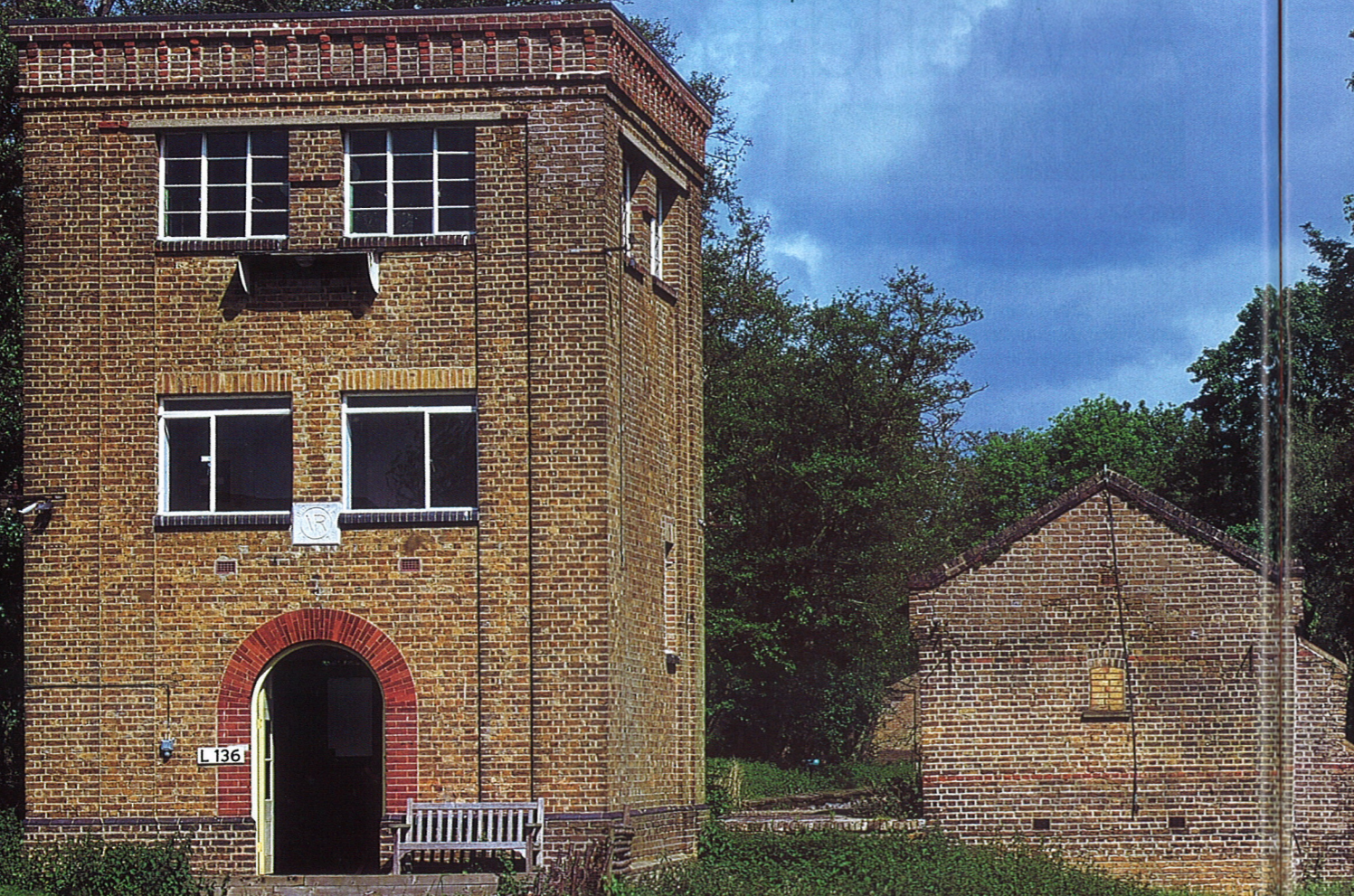
This canal bridge at the Royal Gunpowder Mills dates from 1904.
