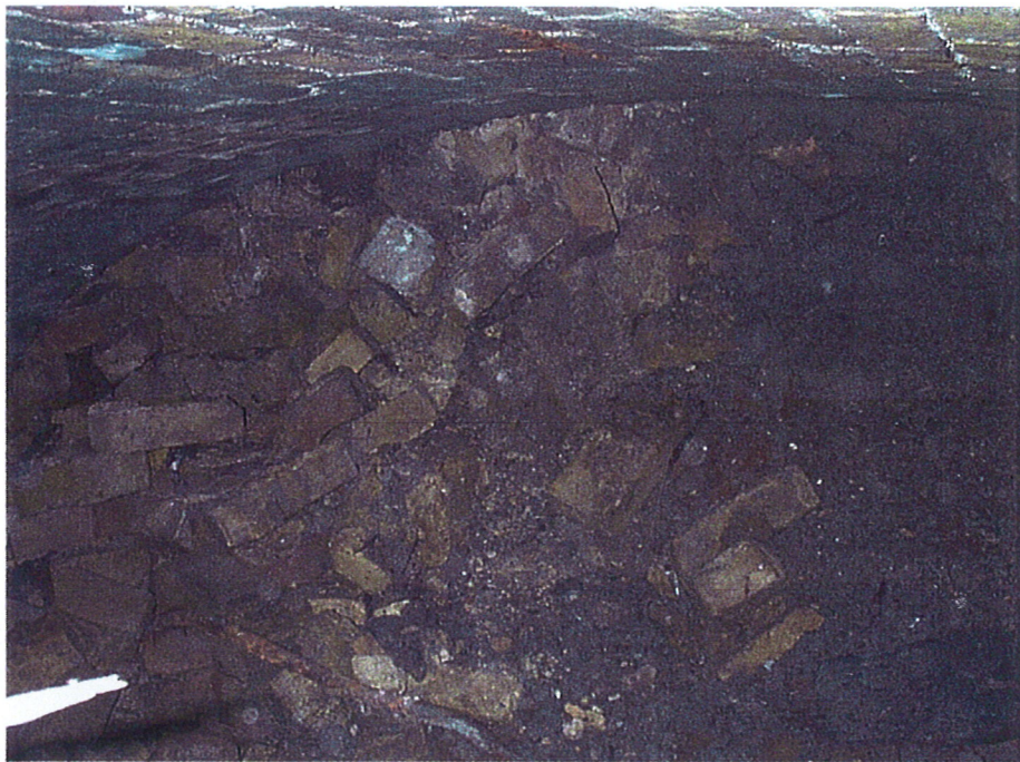
Plate 7. Large Arched Brick Culvert.
