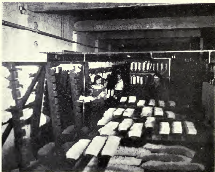
FIG. 72.—VOLKER LIGHTING CORPORATION, LTD. DRYING IMPREGNATED MANTLES.
