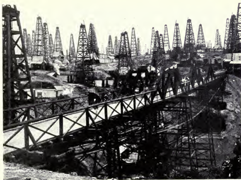
FIG. 94.—IN THE YENOUNGYOUNG DISTRICT (BURMA). KHODARY BRIDGE.
