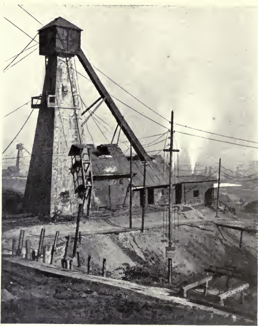
FIG. 89.—GALICIA. DERRICK AND ENGINE SHED.
