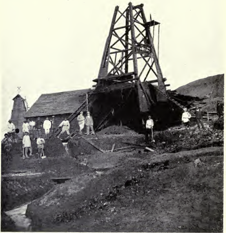
FIG. 92.—GROSNIC (S. RUSSIA) DERRICK AFTER DESTRUCTION BY OIL FOUNTAIN. AKHWERDOFF. No. 7.
