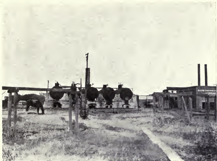
FIG. 97.—LOUISIANA. GENERAL VIEW OF STILLS.
