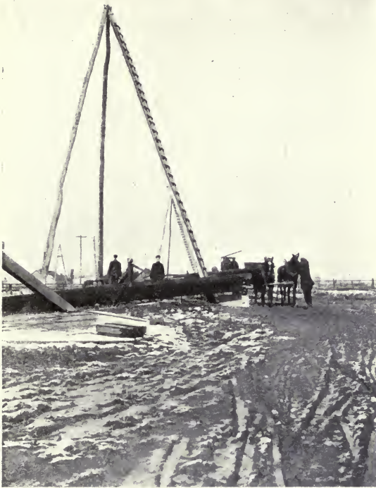
FIG. 77.—PETROLIA, CANADA. THREE-POLE DERRICK USED FOR CLEANING AND REPAIRING PUMPING WELLS.
