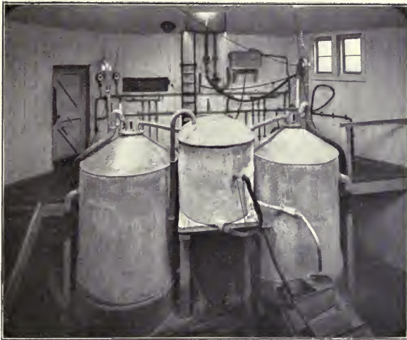
FIG. 139.—NITRATOR-SEPARATORS.
