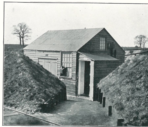
FIG. 131.—MOUNDED HOUSE. COTTON POWDER WORKS.
