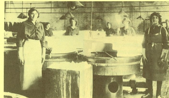
Guncotton nitration by displacement process
