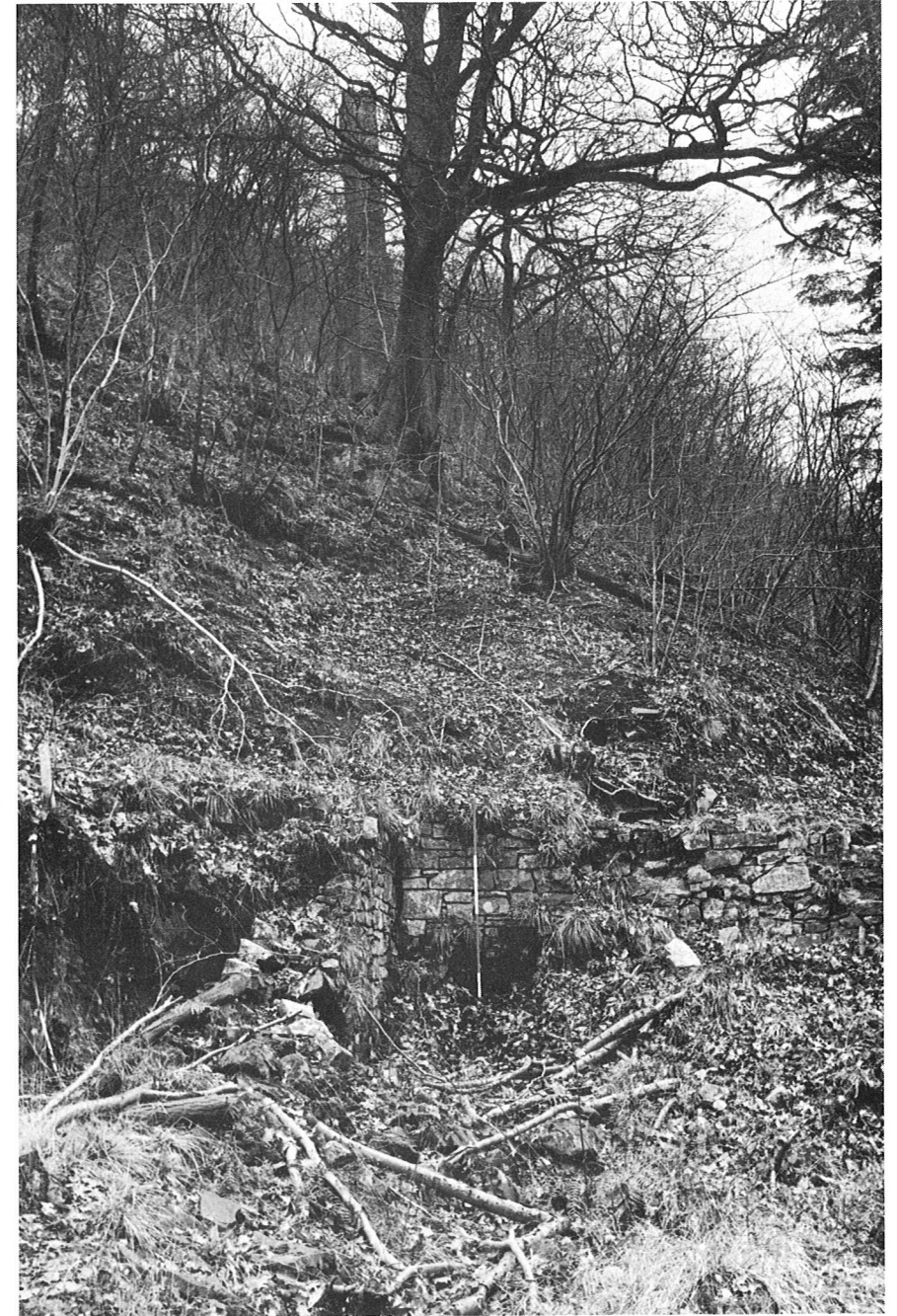
In the foreground is the flue which led from the Boiler House to the stack in the background
