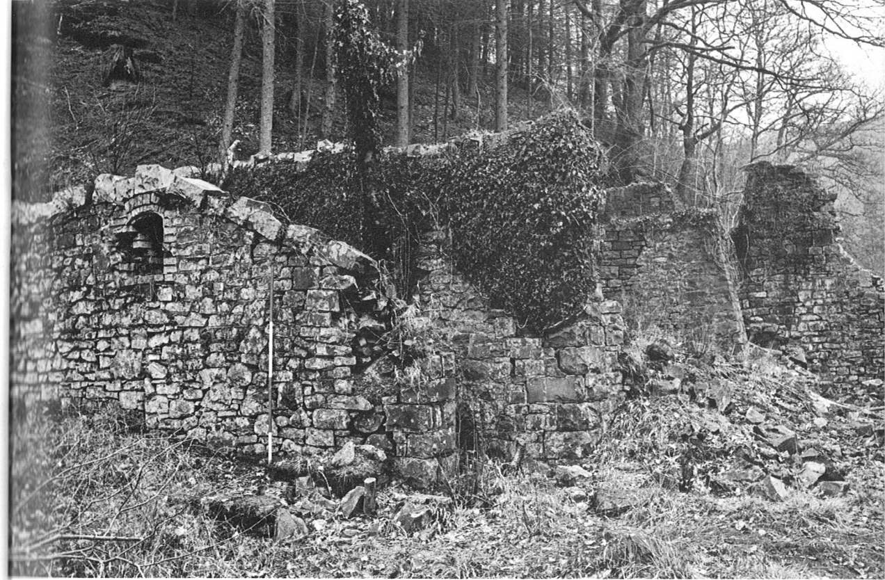
The remaining foundations of the water leat which went over the top of other buildings
