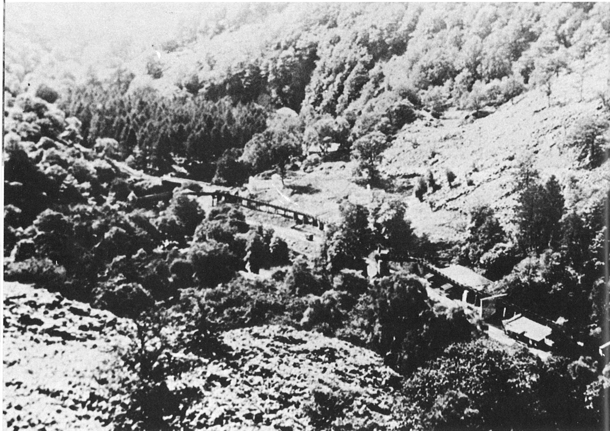
Halfway along the factory showing the upper water leat and the middle bridge across the river. This carried a tramroad which served the buildings on the east side of the river
