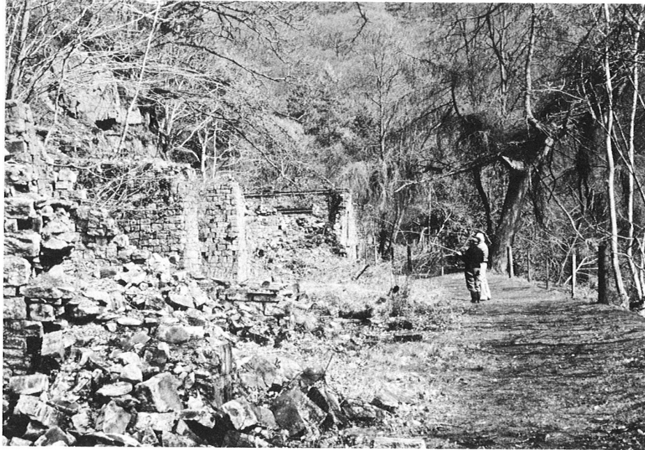
Viewing the old foundations of the water leat from the tramroad
