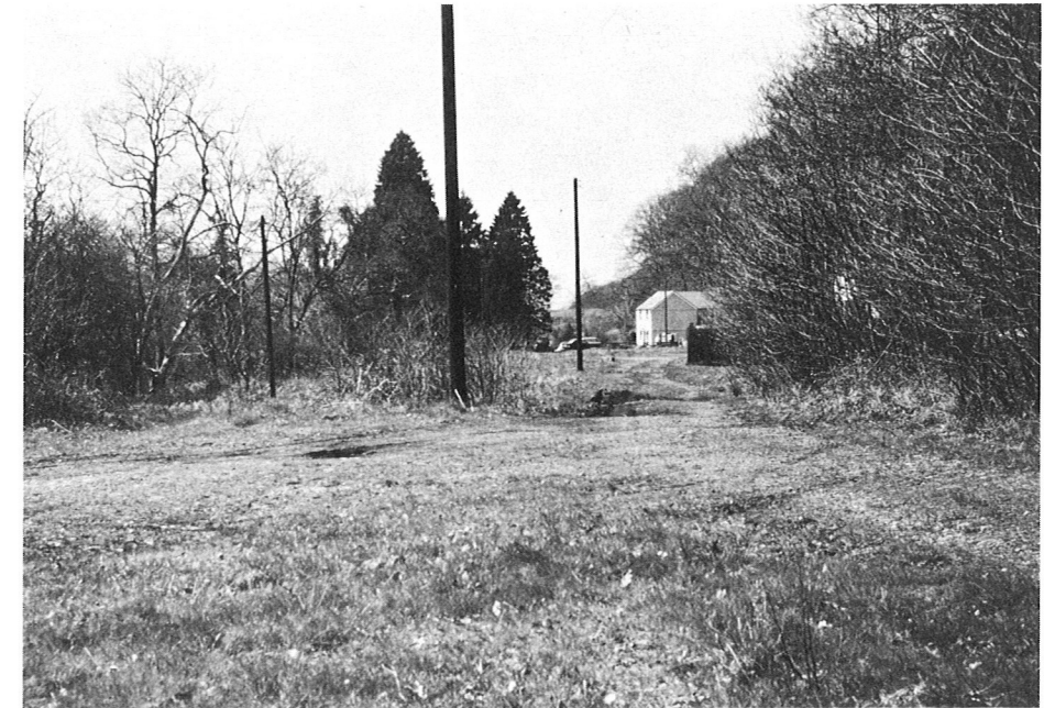
Looking south from the site of one of the old mills. Hollybush Cottage is in the background with Rose Cottage behind the trees
