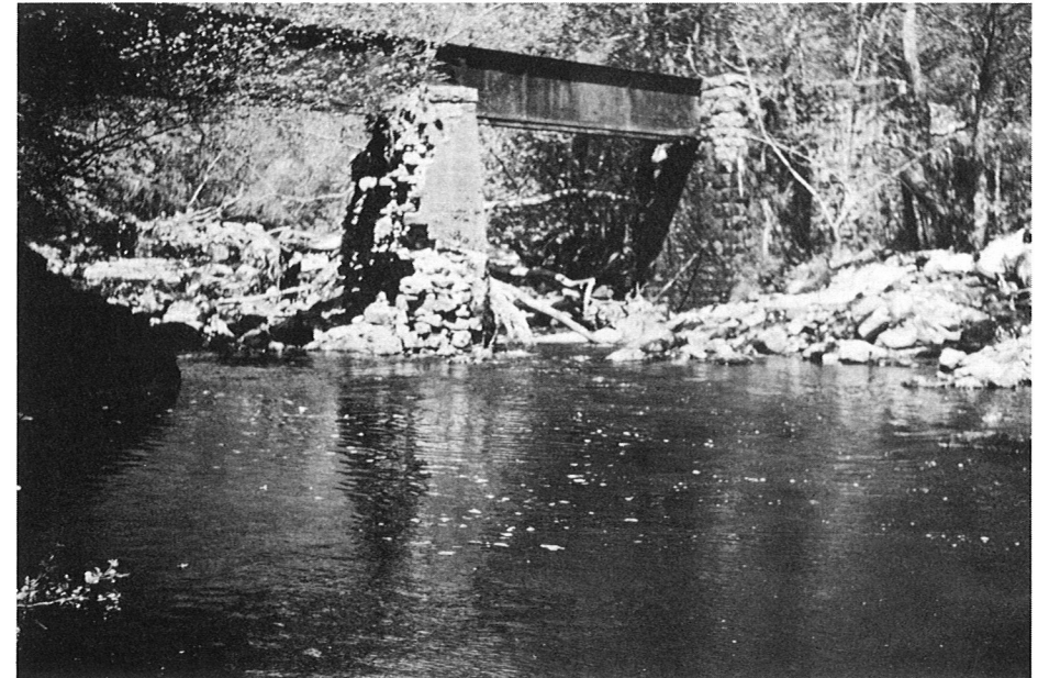
The top bridge which carried the tramroad and water leat. Only the pillars now exist
