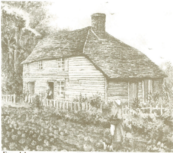
Farm labourers cottages at Woodside, North Weald, as they might have looked in 1886.
