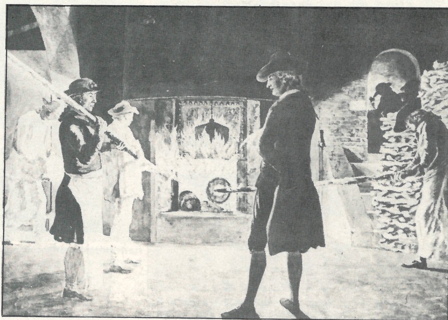
A scene in the furnace room depicting the casting of cannon barrels in the furnace itself
