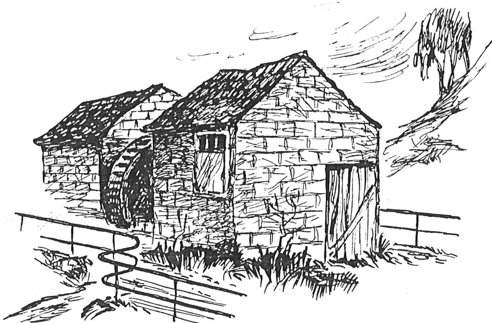
One of the original water wheels dating from 1790. This old paddle wheel drove twin edge-runner grinding wheels, each housed in a separate shed on each side of the wheel.
